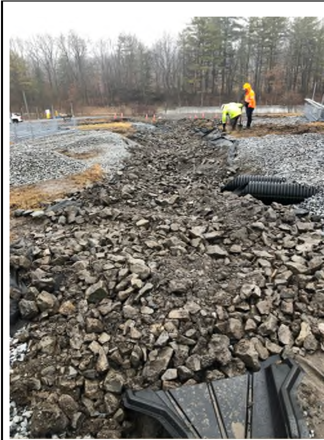
3. Rip-rap placed on geo-textile in down-chute.
