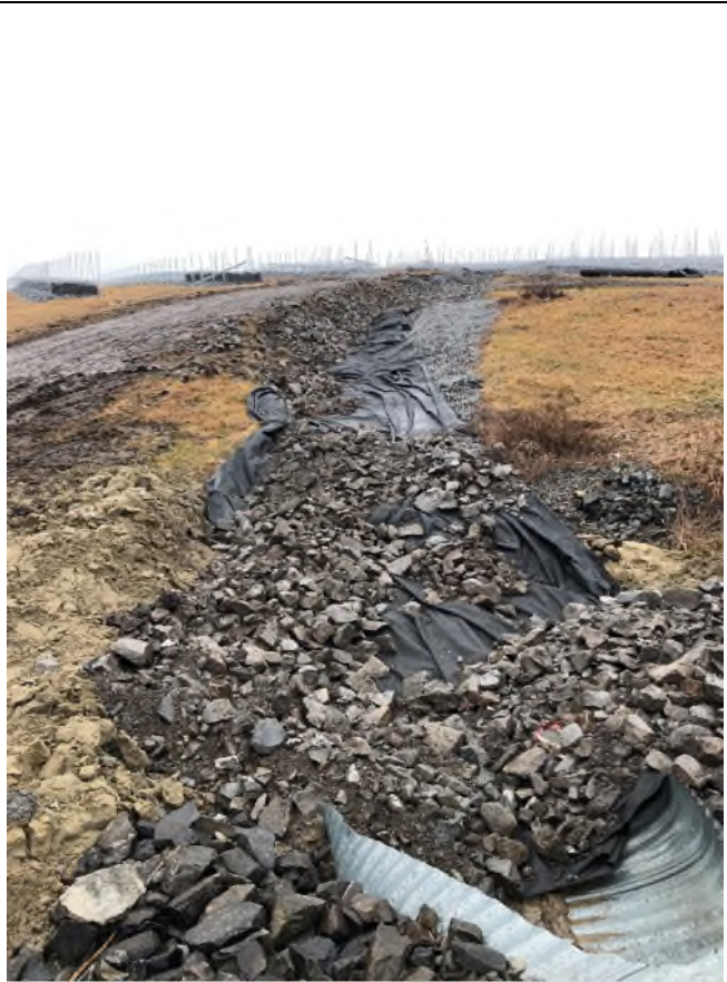
4. View of down-chute from culvert that passes under landfill access driveway.
