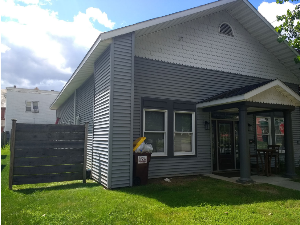
Picture 1: North Side of Building
