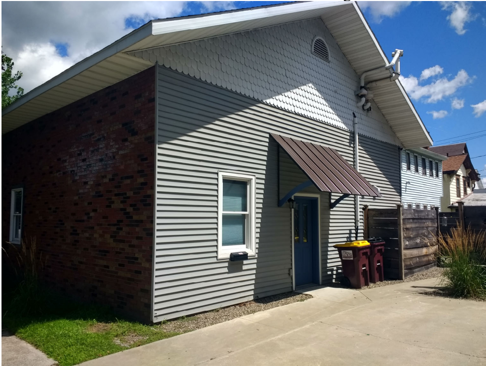
Picture 2: South Side of Building
