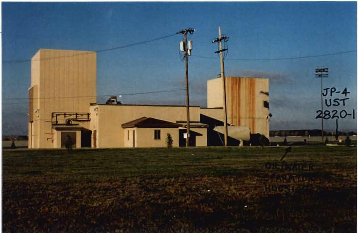
PHOTO 1 - A westward view of the east side of the Jet Engine Test Cell (Building 2820).
