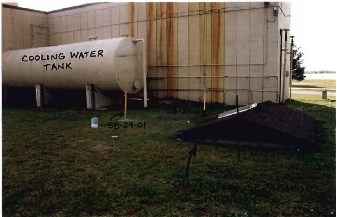
PHOTO 2 - A southwestward view of the northeast end of Building 2820 showing the oil/water separator housing, the cooling water tank, and two soil boring locations (orange-flagged stakes) .
