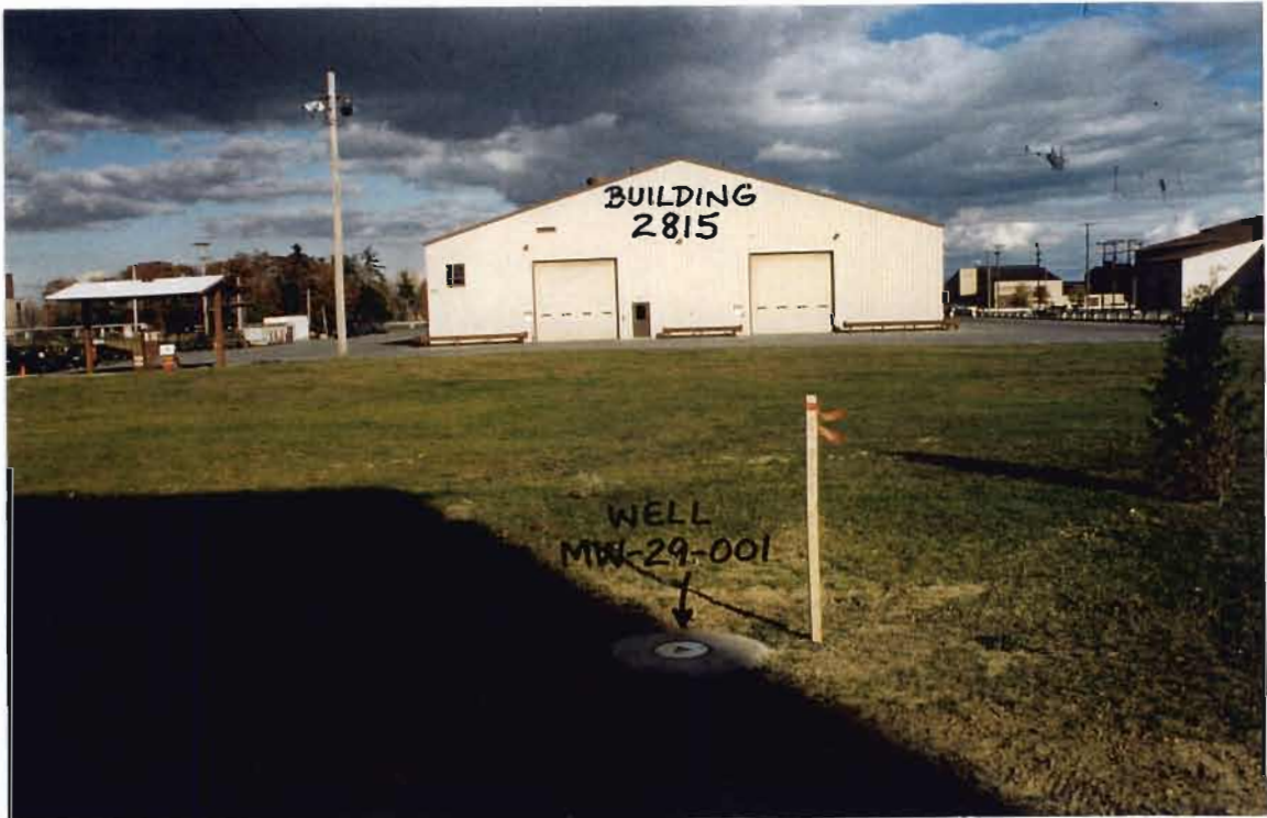
PHOTO 4 - An eastward view of well MW-29-001 with Building 2815 (Aerospace Ground Equipment Facility) in the background.
