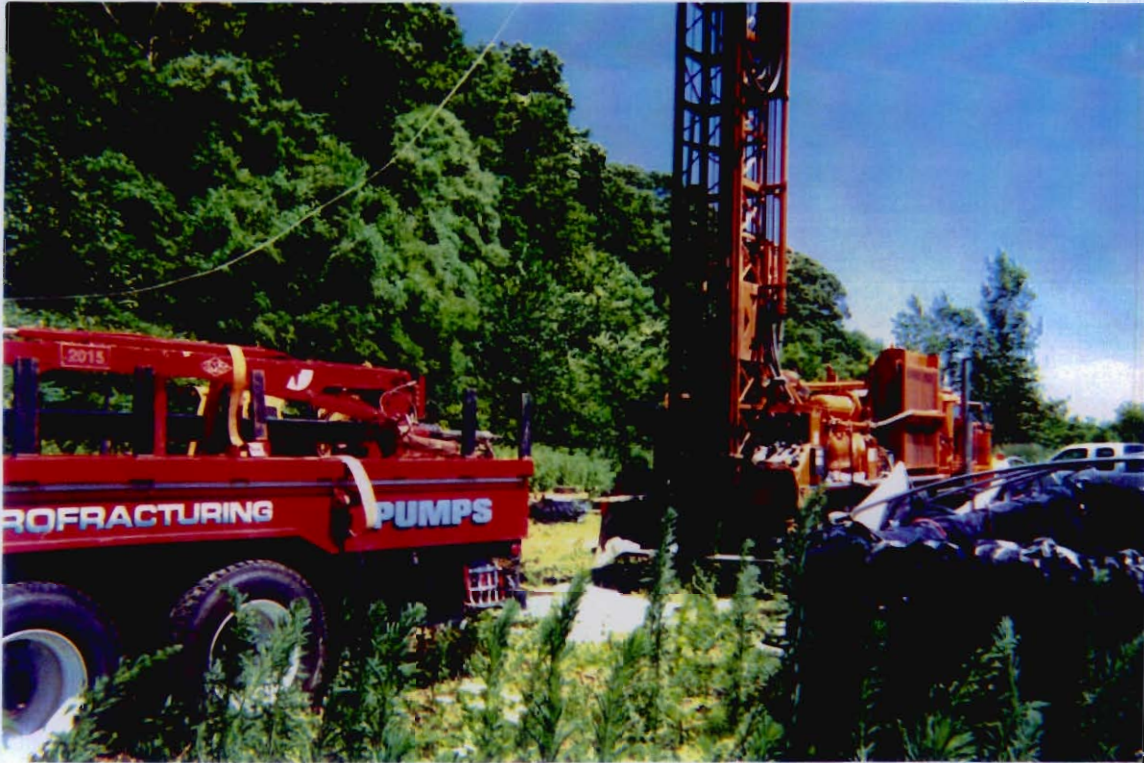
Description: Drill rig set up on PMW-7. Date: July 5, 2000
