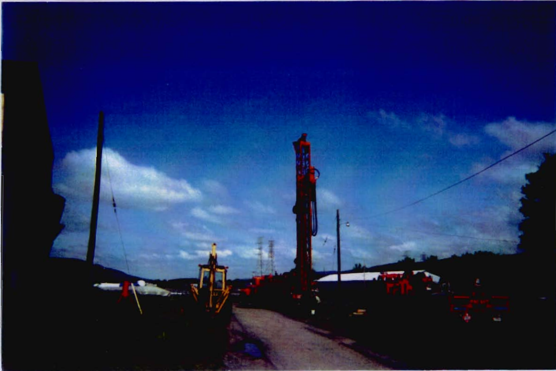
Description: Drill rig set up on PMW-3. Date: June 7, 2000
