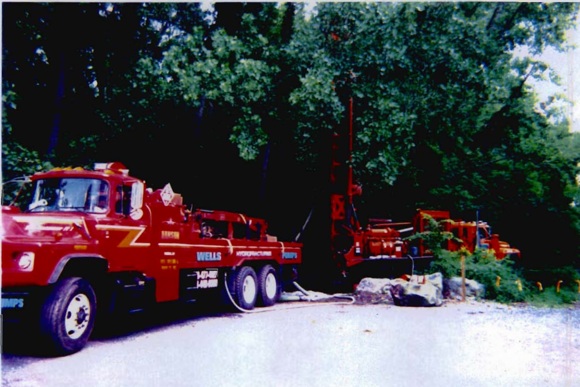
Description: Drill rig set up on PMW-6. Date: June 29, 2000
