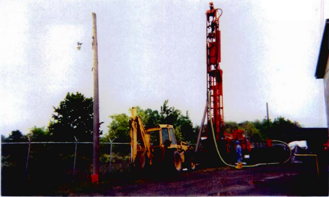
Description: Drill rig set up on PMW-1. Date: May 22, 2000
