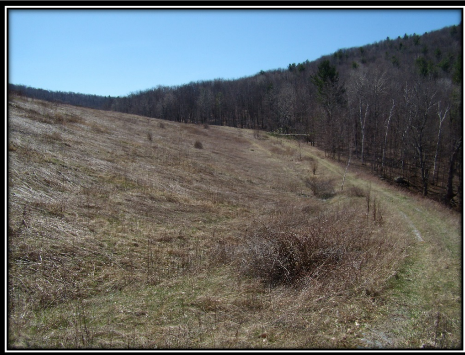
Photos 12 and 13: Vegetation is growing within all of the stormwater features. This could eventually lead to erosion and slope stability issues if not addressed.
