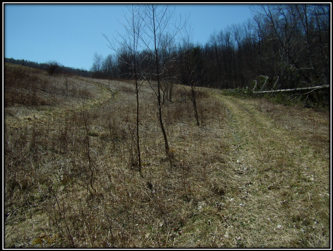
Photos 12 and 13: Vegetation is growing within all of the stormwater features. This could eventually lead to erosion and slope stability issues if not addressed.
