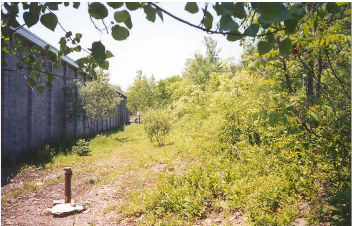
Northeast of Building
