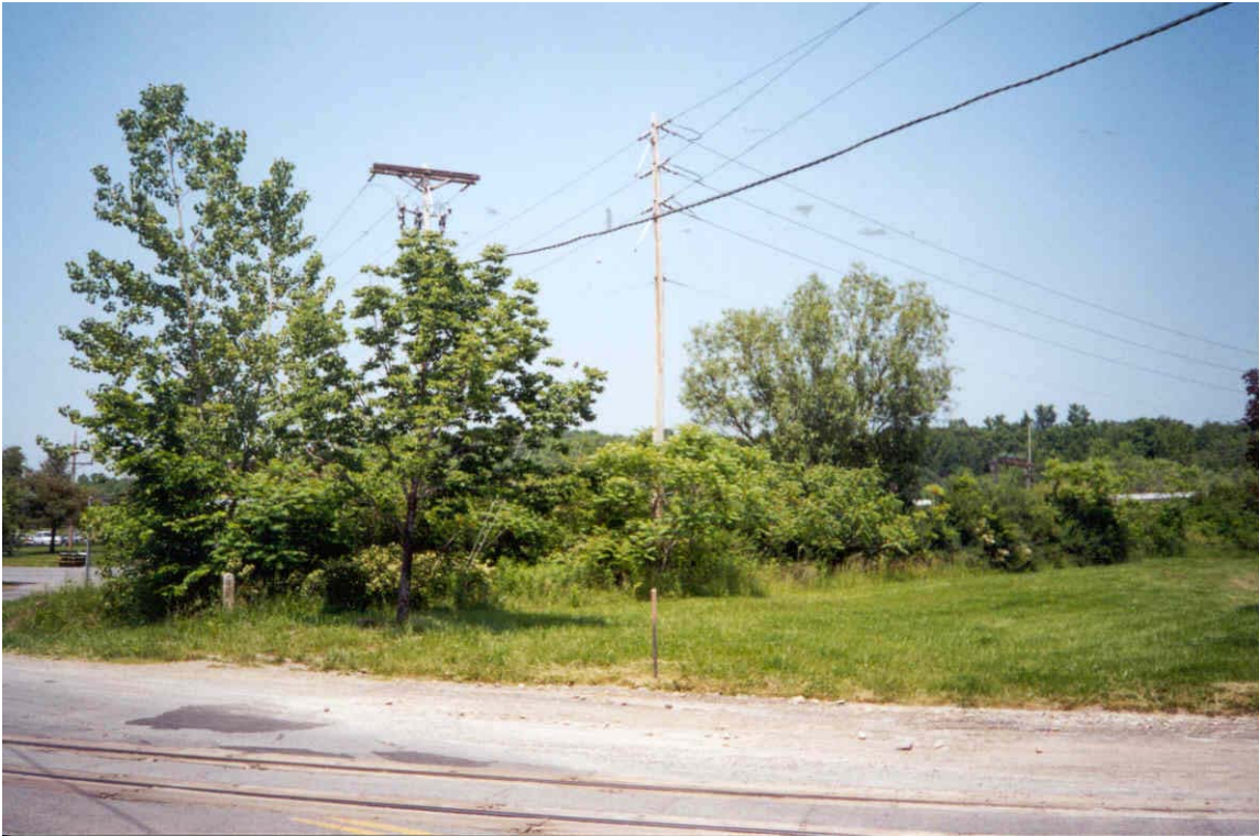
Ditch at Edson Street (North)
