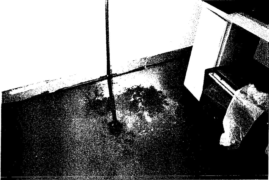
PHOTO 5. SB-7 installed in vacant tenant space adjacent to the west of the Guilderland Dry Cleaners tenant space.
