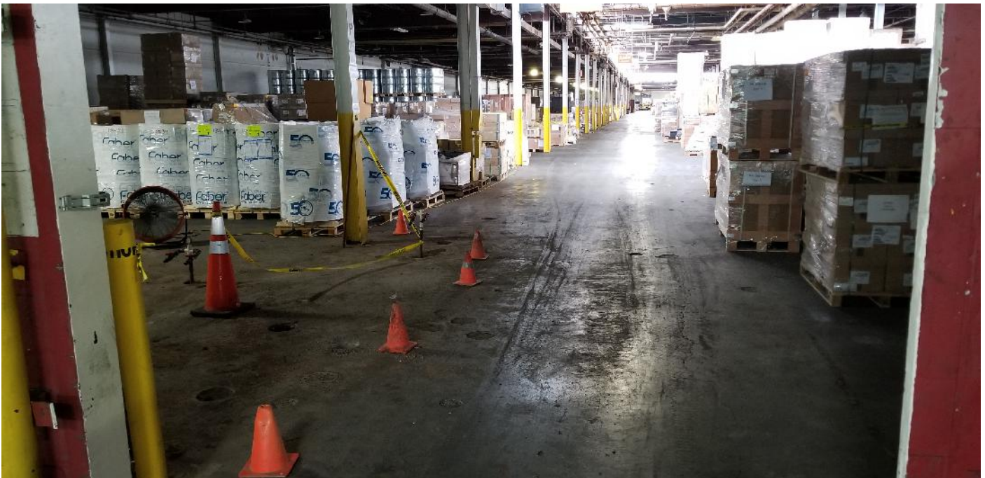
Picture 6: Building #58 ISCO injection area//forklift path indoor air monitoring area (view looking south)
