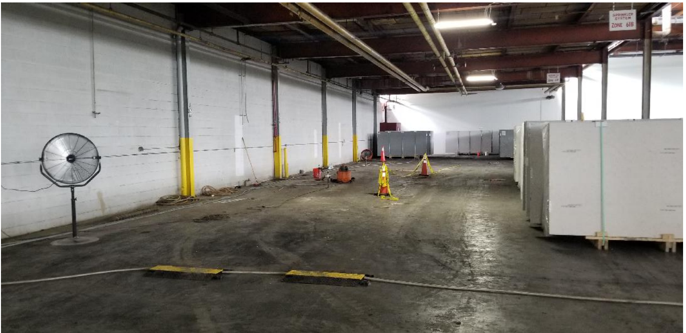
Picture 4: Building #61 ISCO injection area/exclusion zone indoor air monitoring area (view looking east)
