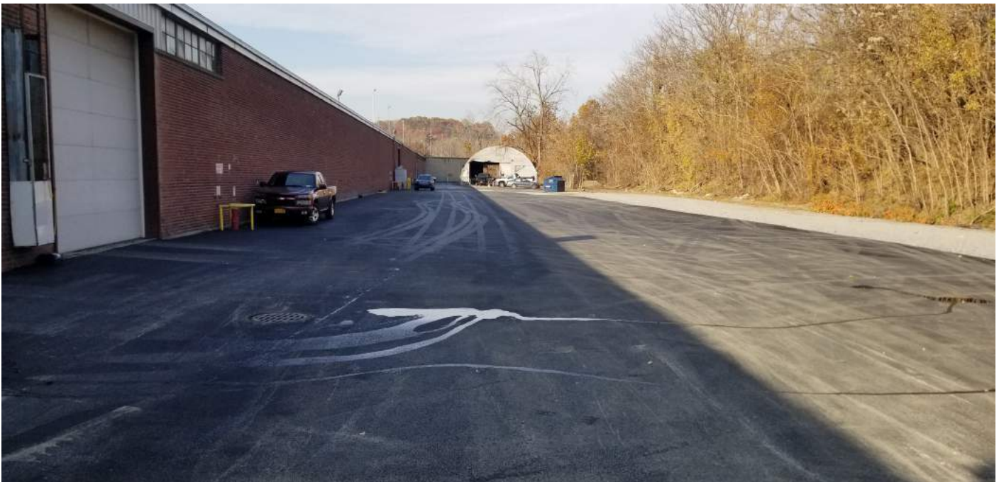
Figure 6. Paved parking area north of Building #61 (view looking west).
