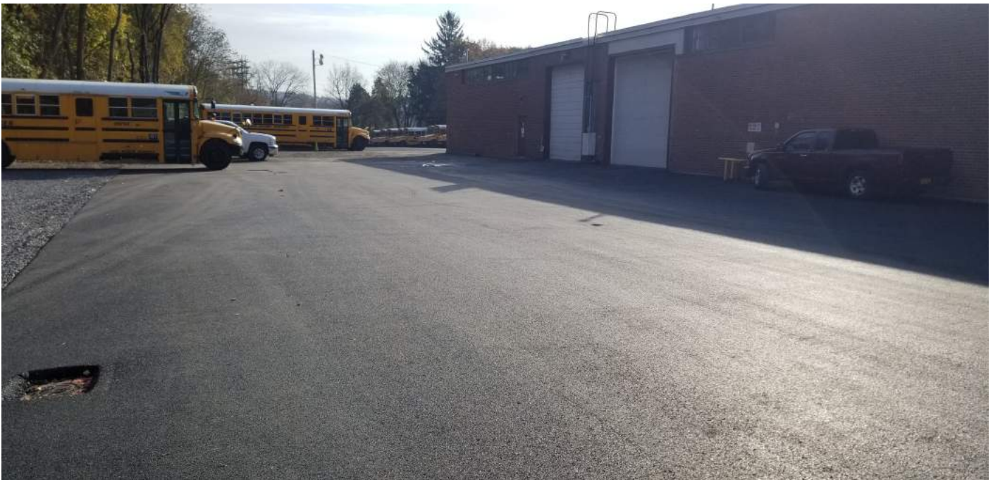
Figure 4. Paved parking area north of Building #61; monitoring well MW-27 in foreground (view looking east).
