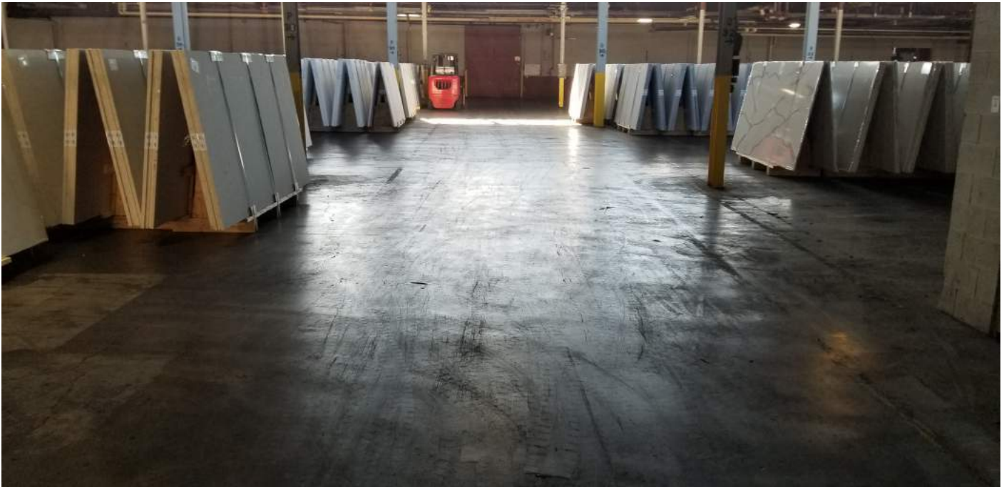
Figure 13. Concrete slab inside the northern portion of Building #61 (view looking south)
