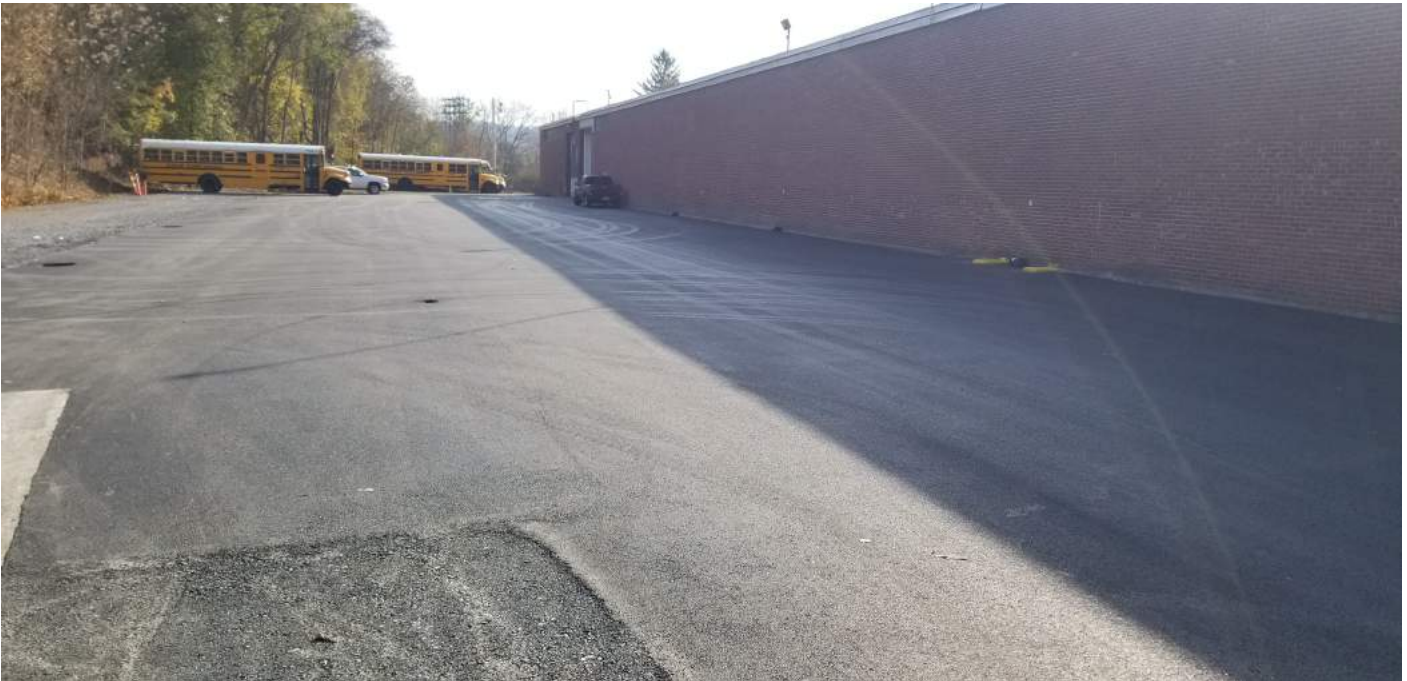
Figure 2. Paved parking area north of Building #61 (view looking east).
