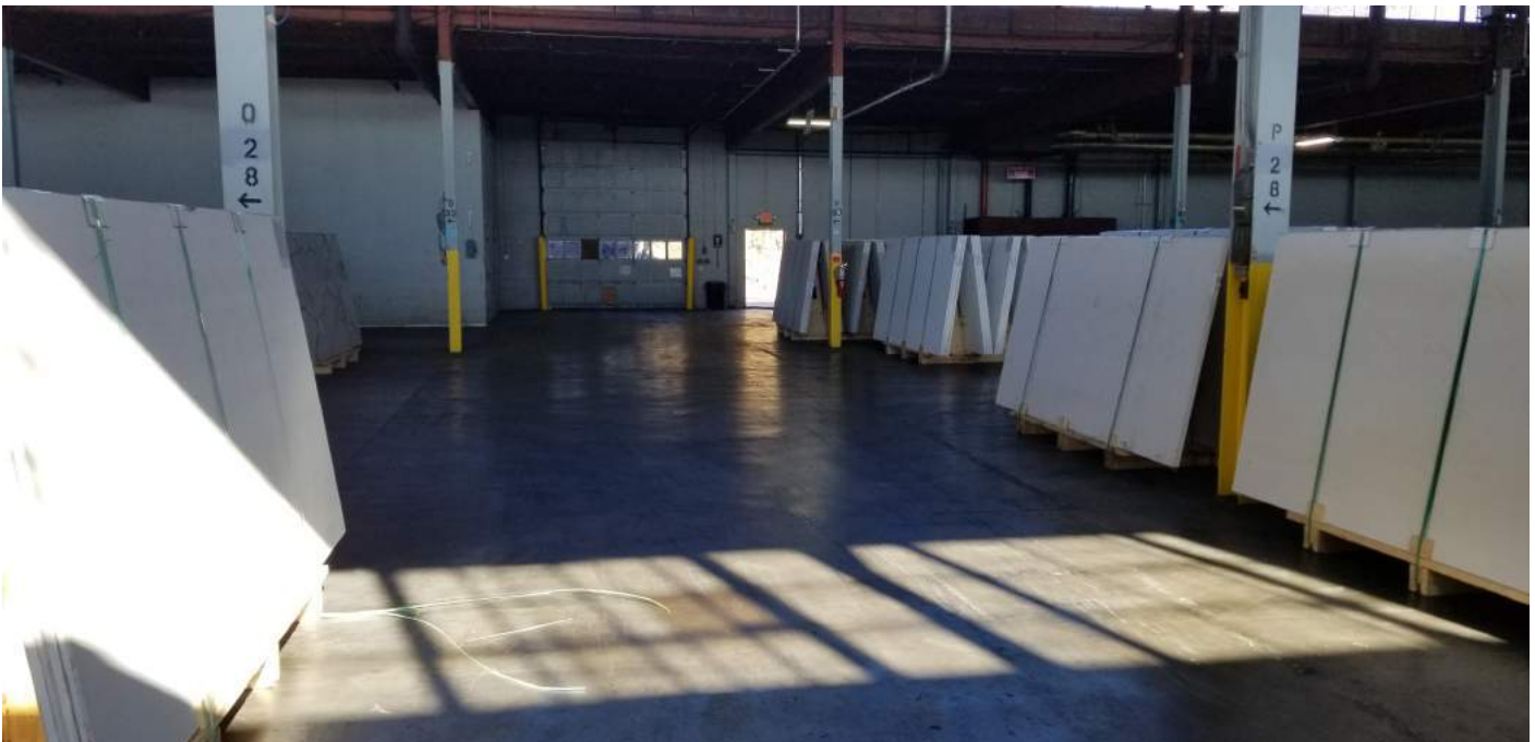
Figure 14. Concrete slab inside the northern portion of Building #61 (view looking north)
