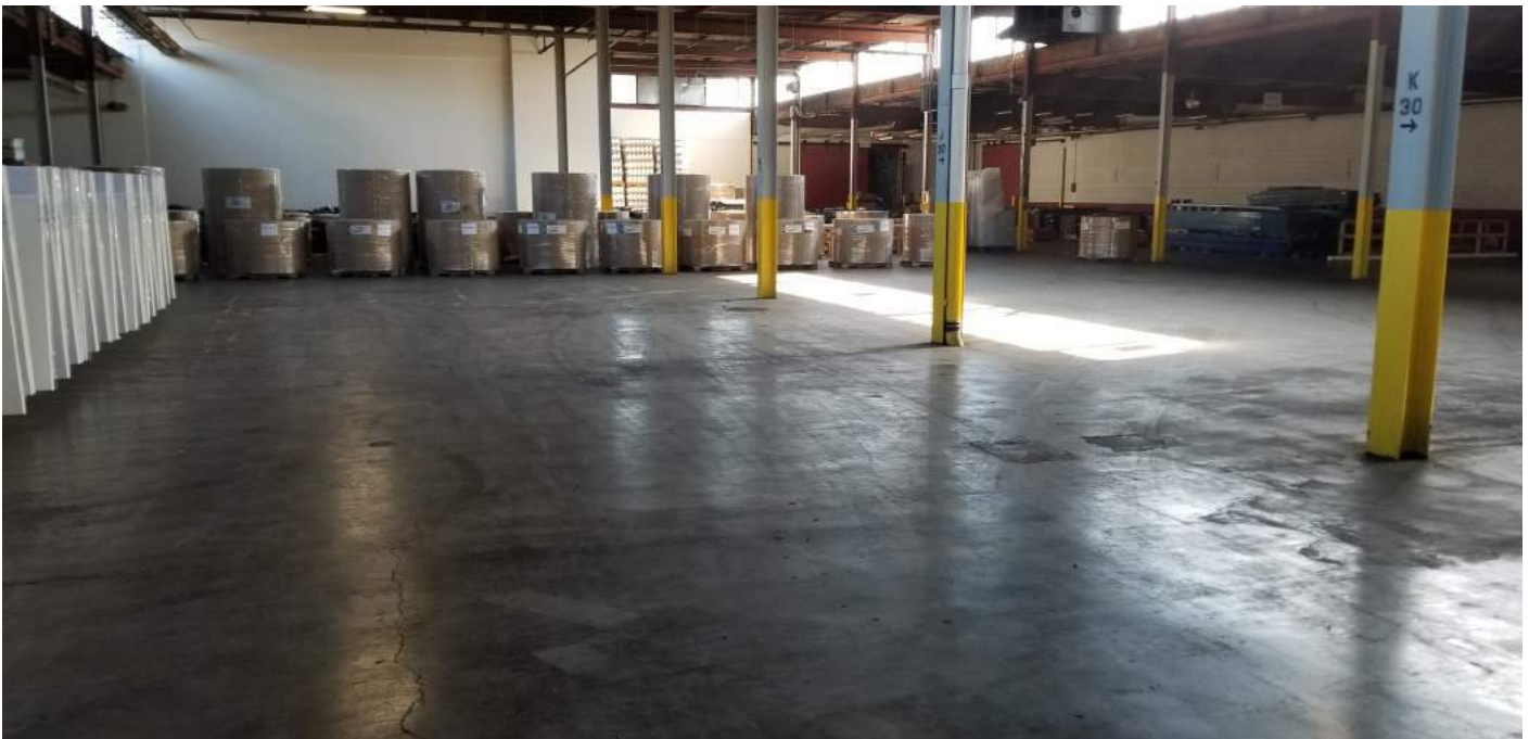
Figure 18. Concrete slab in Building #61 (view looking east)
