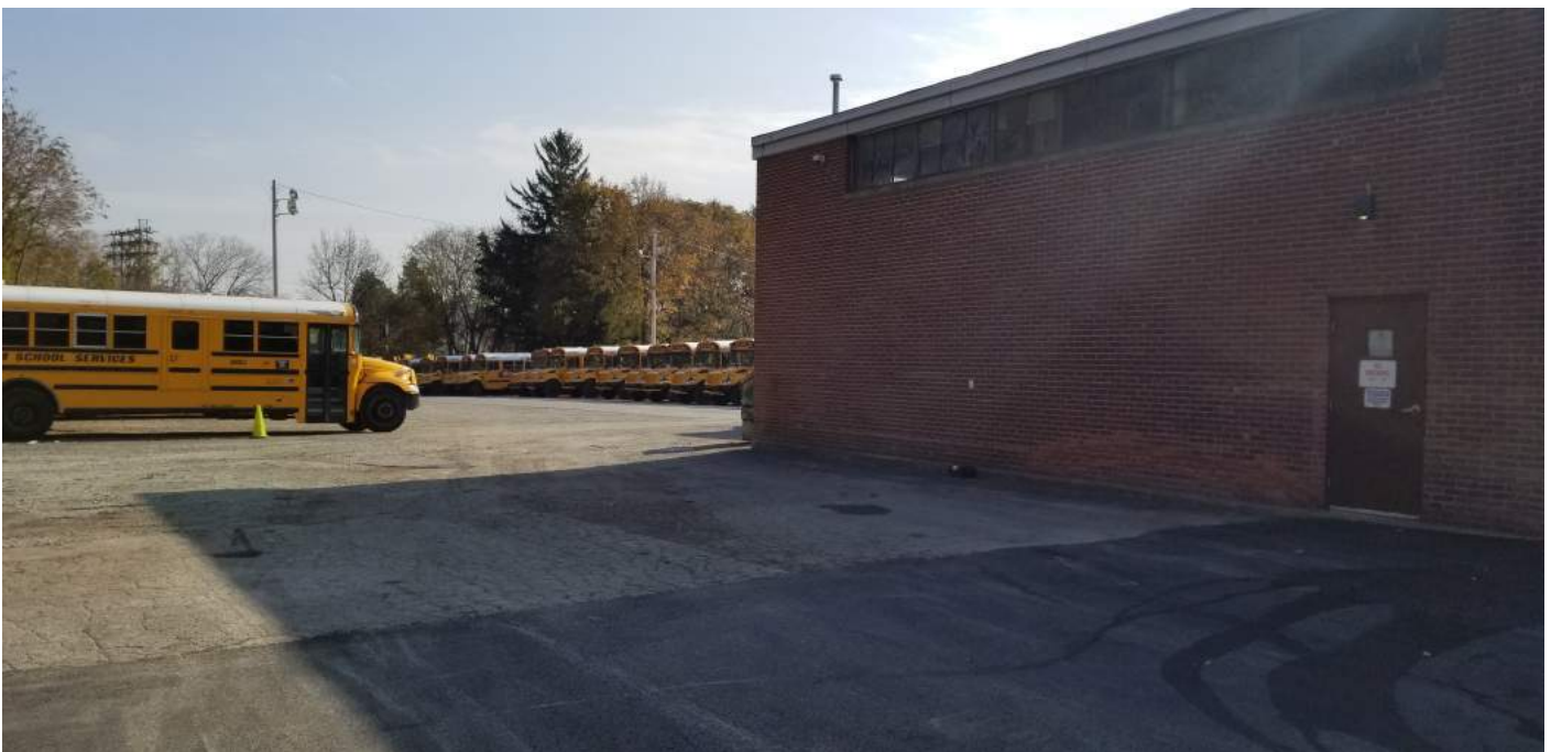
Figure 12. Eastern end of paved area proximal to Durham Bus garage (view looking southeast)
