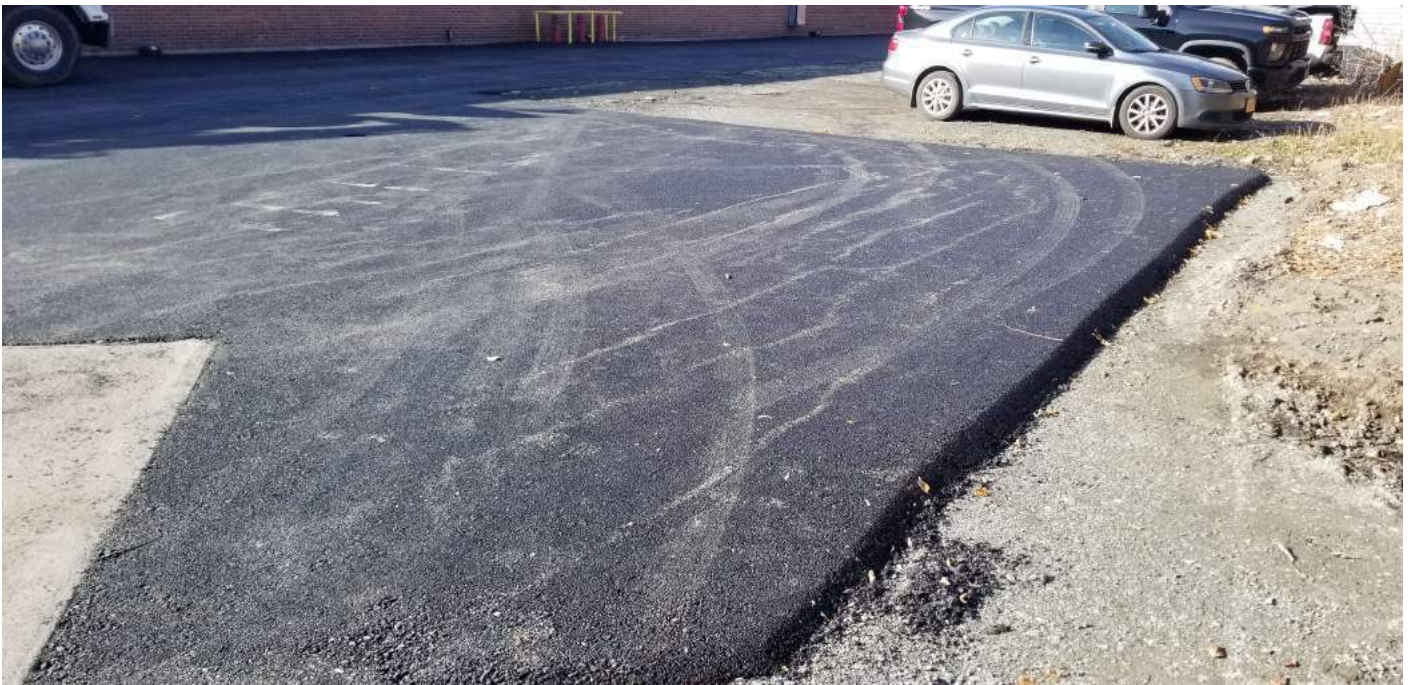
Figure 11. Northwestern corner of paved area (view looking southwest)
