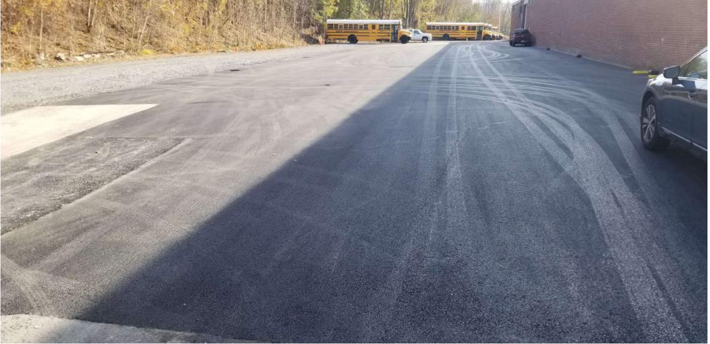
Figure 1. Paved parking area north of Building #61 (view looking east).
