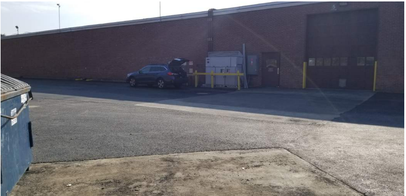
Figure 10. Paved parking area north of Building #61; western end of Environmental Easement (view looking southeast)
