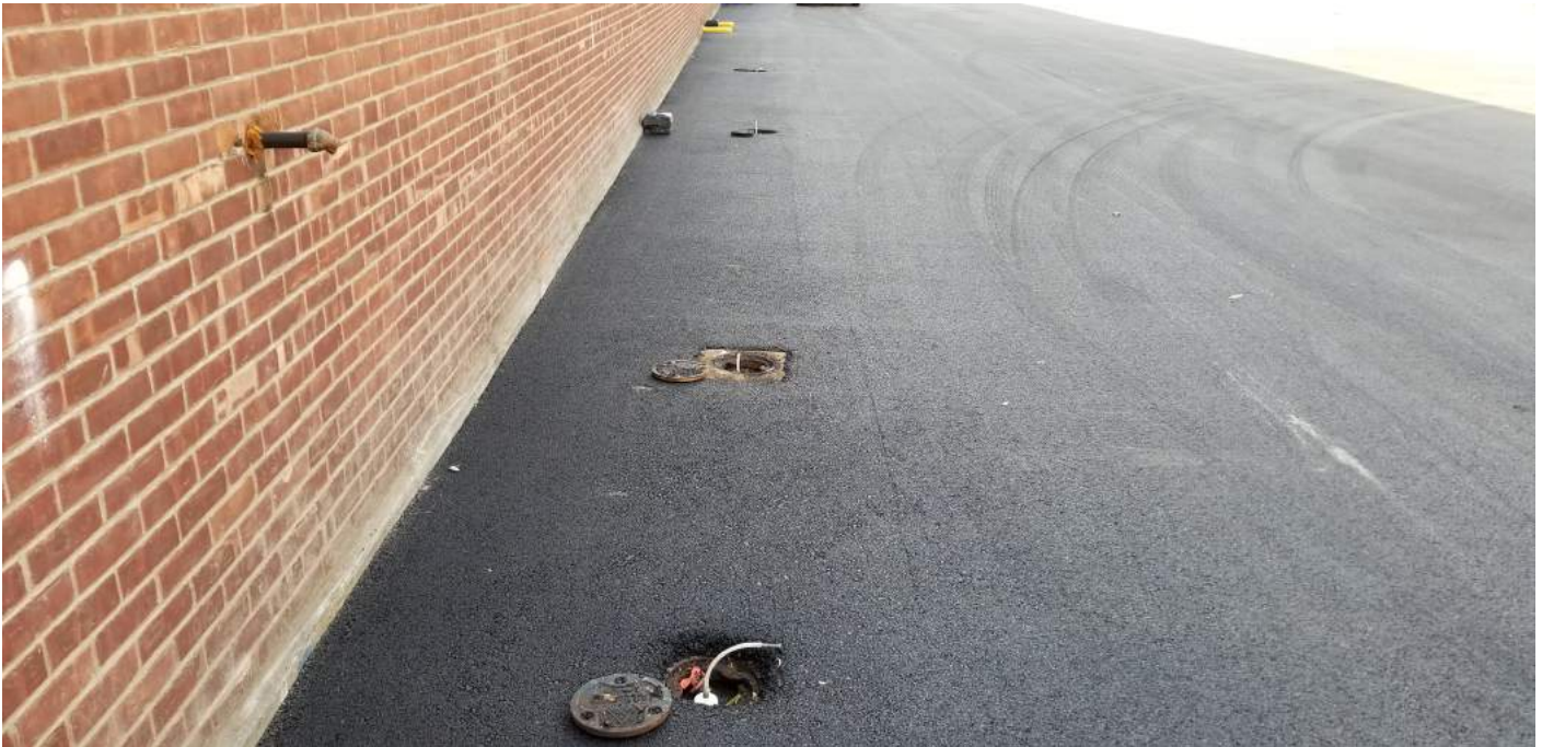
Figure 9. Paved area north of Building #61; monitoring well MP-25 in foreground (view looking west).
