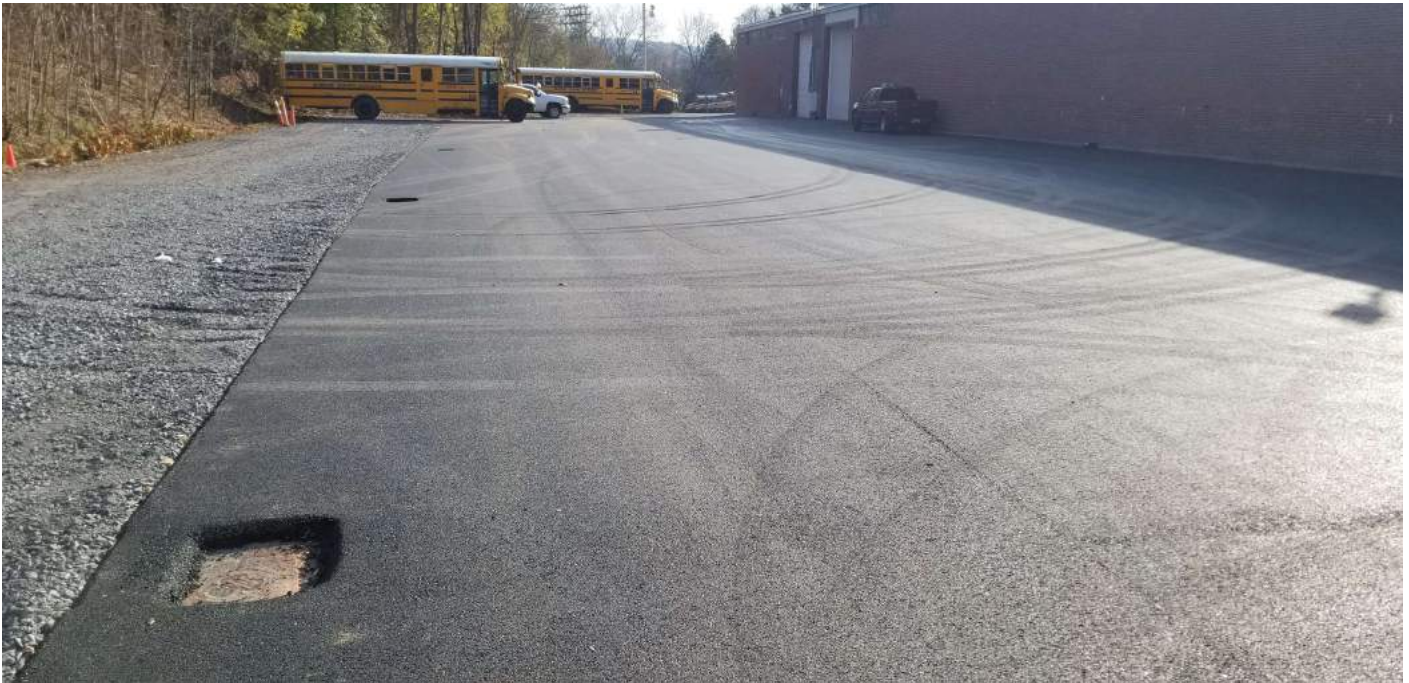
Figure 3. Paved parking area north of Building #61; monitoring well MW-25 in foreground (view looking east).
