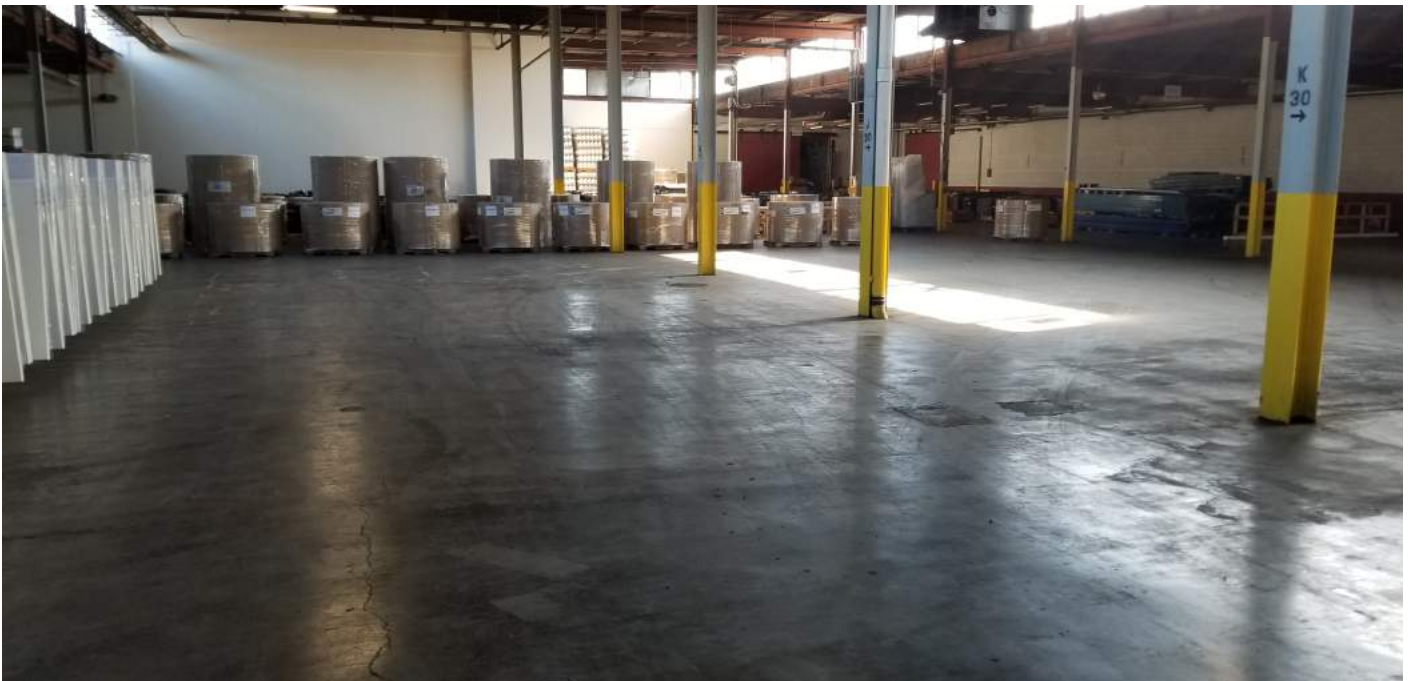
Figure 18. Concrete slab in Building #61 (view looking east)
