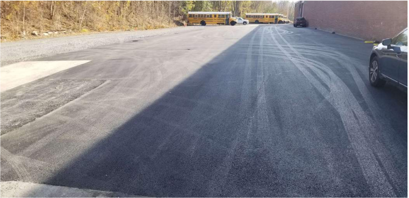
Figure 1. Paved parking area north of Building #61 (view looking east).
