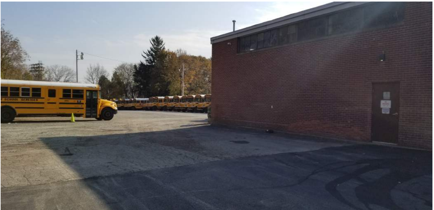
Figure 12. Eastern end of paved area proximal to Durham Bus garage (view looking southeast)
