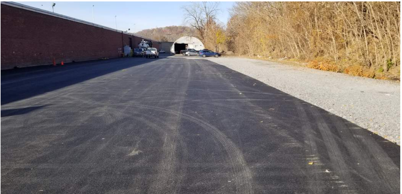
Figure 8. Paved parking area north of Building #61 (view looking west)
