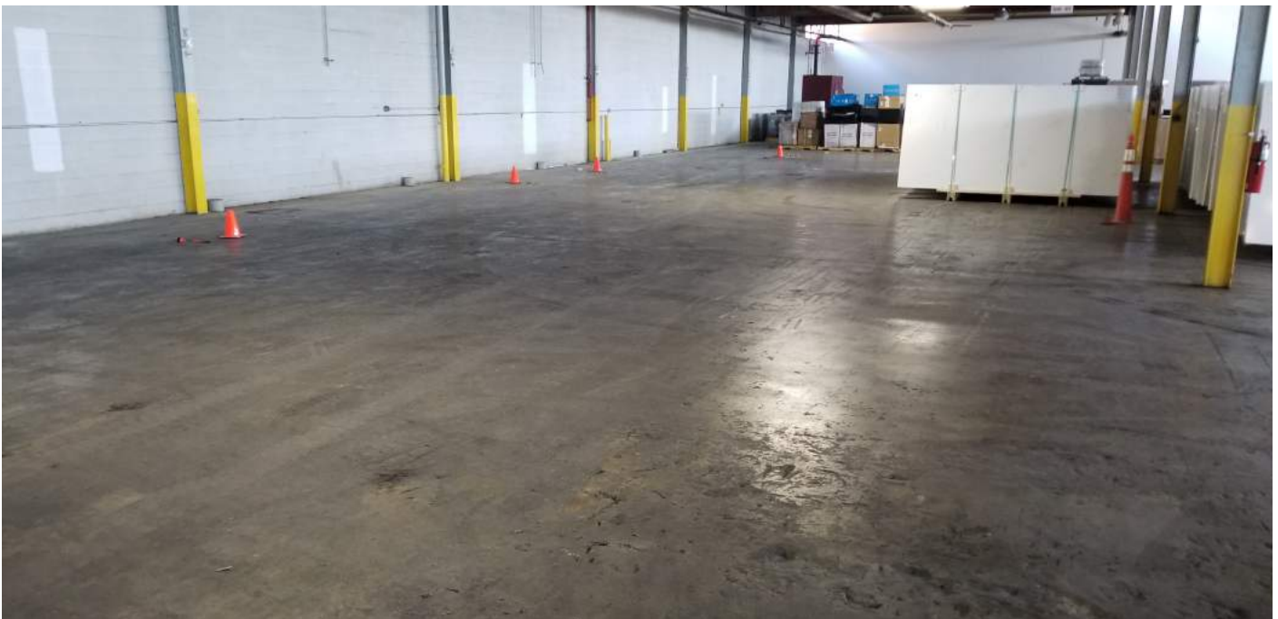
Figure 16. Concrete slab inside the northern portion of Building #61; traffic cones at monitoring wells MW-20, MP-26, MP-27, and MP-28 (left to right) (view looking northeast)
