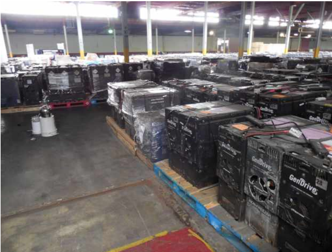
Picture 7: Plug Power “Gen Drive” Forklift Batteries proximal to VMP-3 (PID: 975 – 1,100 ppbv).
