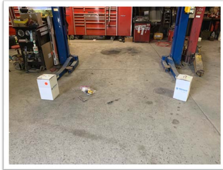
8. A View from the Interior Portion of the Site (SVE Wells Location - Sub-Slab)
