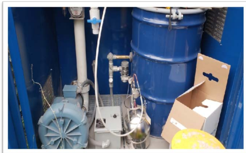
2. Air Sampling at the Discharge of the Blower by Using Suma-Canister
