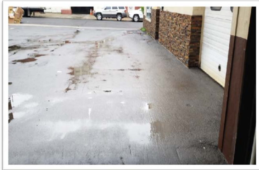
11. A View from the Exterior Portion of the Site (Sub-Slab Area)
