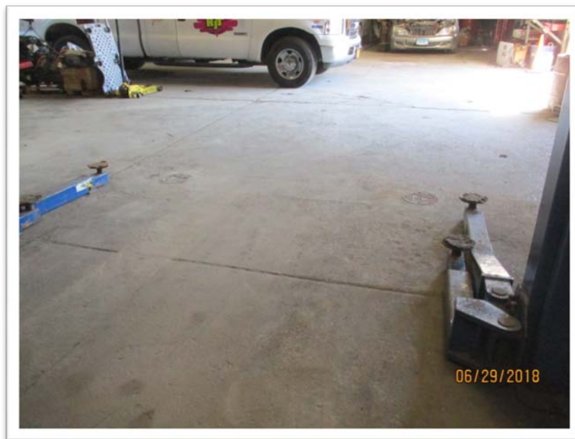
12. A View from the Interior Portion of the Site (SVE Wells Location - Sub-Slab)
