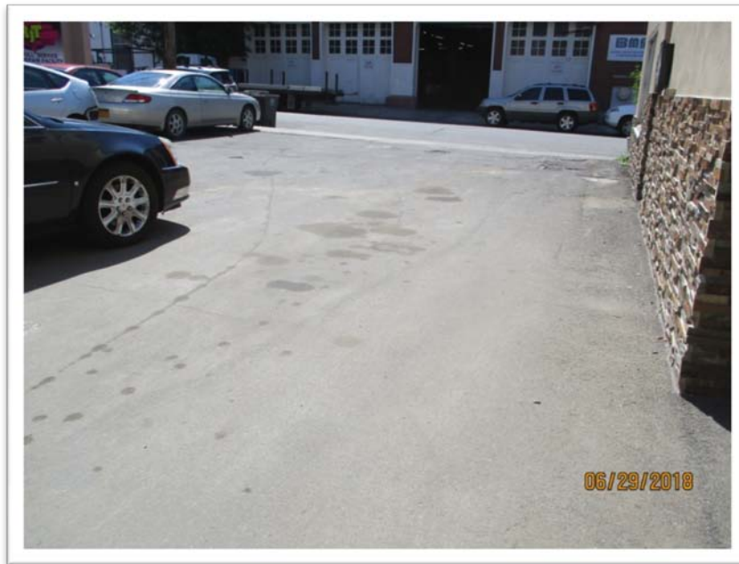
11. A View from the Exterior Portion of the Site (Sub-Slab Area)
