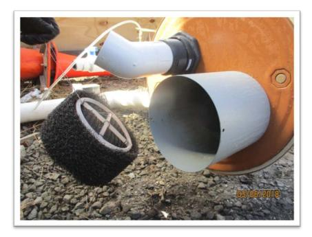
12. Cleaning the Filter/Demister Assembly inside the Knock out Drum
