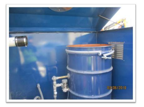
11. System Maintenance by Removing the Cover of the Knock out Drum
