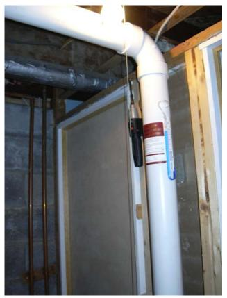
**Description:** View of the U-tube manometer and labeling on the vertical PVC suction piping in the utility room.
