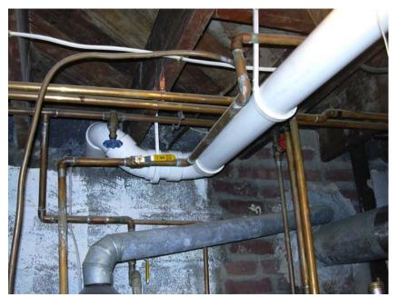
**Description:** View of the system piping (3-inch diameter white PVC pipe) exiting the building along the north wall.
