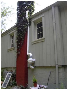
**Description:** View of the fan and exhaust piping along the north side of the building.
