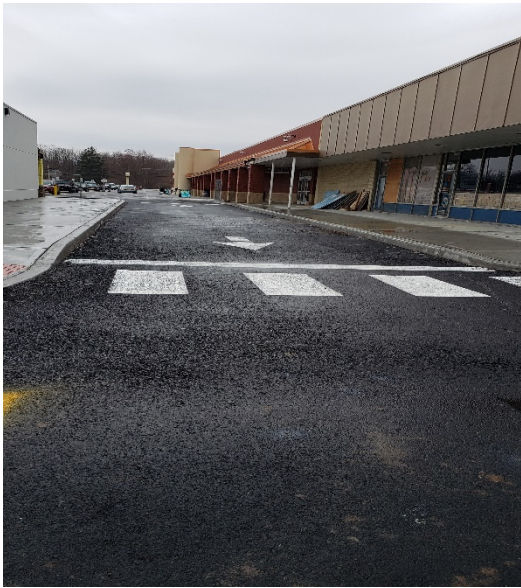
SITE CONDITION PRIOR TO DRILLING
