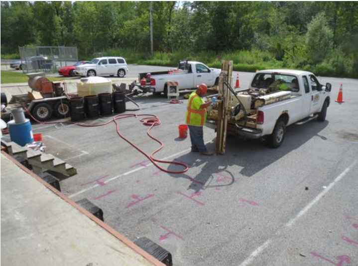
Photograph No. 3: Injecting bioremediation solution at IP2. Purple painted lines indicate location of subsurface anomalies.
