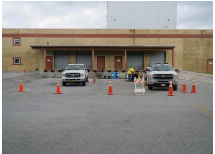
Photograph No. 2: AOC-6 bioremediation application work area.
