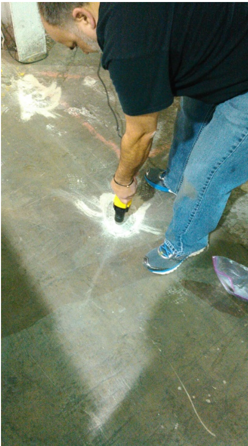
Photo No. 7: Creating SSVI sample Port LCS-1 in Rental Space A2, 24 Seven.
