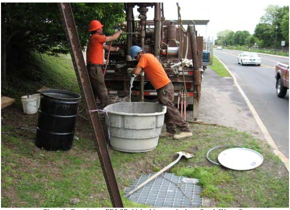
Photo 9: Grouting at PDI-SB-11 looking north along South Water St.
