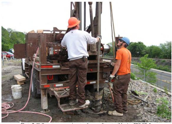
Photo 7: Hollow stem auger rig setup for sampling at soil boring PDI-SB-5.
