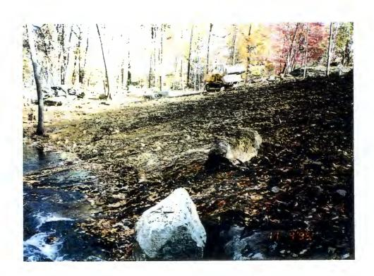
TEMPORARY REMOVAL OF SILT FENCE AND RE-GRADE AT THE TOE BOUNDARY
