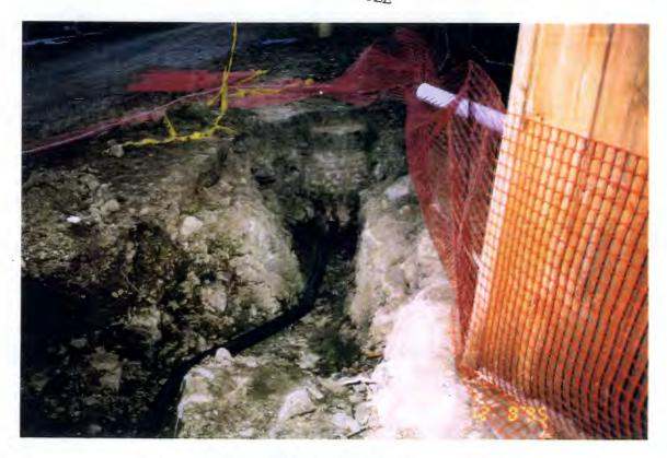
CONNECTING CATCH BASIN TO THE SANITARY MANHOLE WITH SIX INCH FLEXIBLE PIPE
