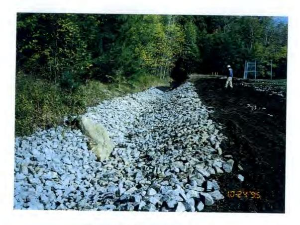
PLACING RIPRAP IN THE NORTH END OF THE DRAINAGE SWALE
