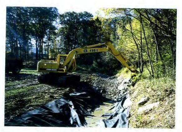
PLACING RIPRAP IN SOUTH END OF DRAINAGE SWALE
