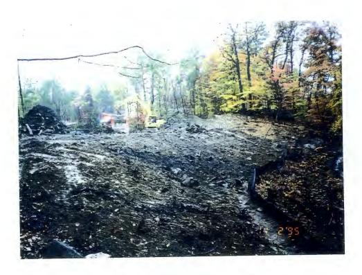
MATERIAL REMOVAL AND SLOPE RE-GRADE
