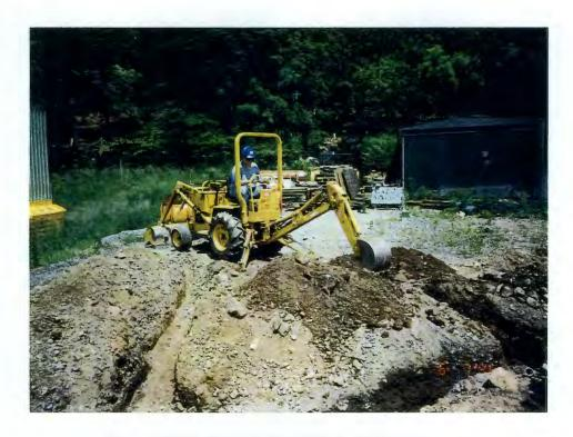
EXCAVATING TRENCH FOR NEW ELECTRIC LINE AND MANWAY
