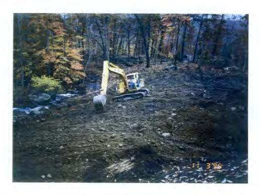
TEMPORARY REMOVAL OF SILT FENCE AND RE-GRADE AT TOE BOUNDARY
