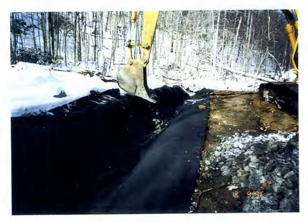
PLACING 6-12 INCH RIP RAP INTO GEOTEXTILE LINED TRENCH
