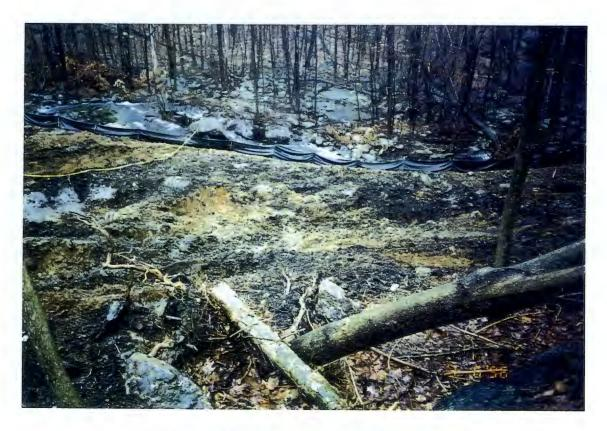
OVER EXCAVATED A 12'x12'x1' VOLUME AROUND CONFIRMATORY SOIL GRAB SAMPLE MF-C1-3
