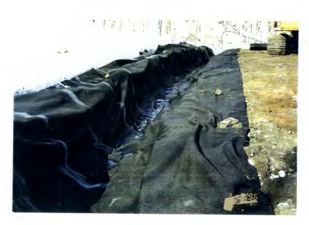
CONSTRUCTING THE FRENCH DRAIN USING 6-12 INCH RIP RAP WRAPPED IN GEOTEXTILE FABRIC
