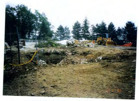
BACKFILLING THE BASEMENT WITH BRICK, CONCRETE AND FILL MATERIAL
