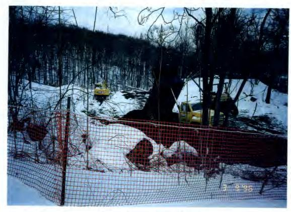
TRANSPORTING "CLEAN" PROCESSED SOIL FROM CRAGSTON LANDFILL TO MORGAN FARM LANDFILL FOR BACKFILL
