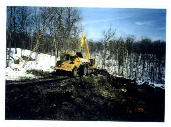
LOADING EXCAVATED LANDFILL MATERIAL INTO ARTICULATED DUMP TRUCK
