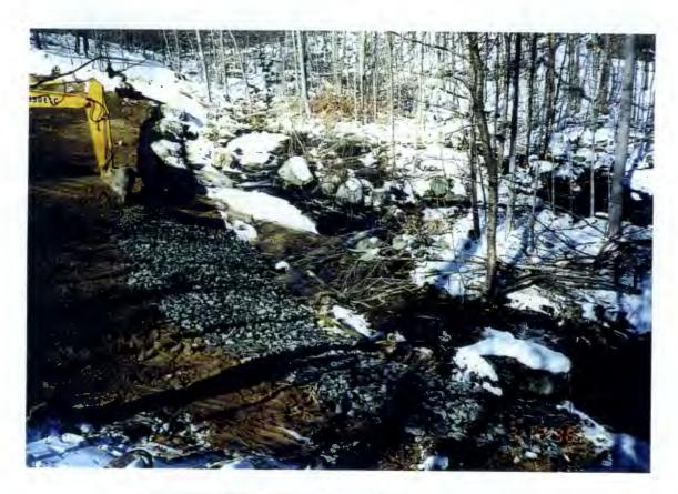
PLACING RIP RAP ON TOP OF GEOTEXTILE FABRIC
