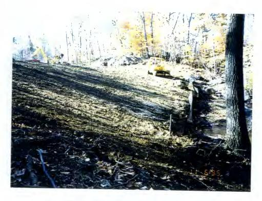
RE-INSTALLATION OF SILT FENCE (90% COMPLETE)
