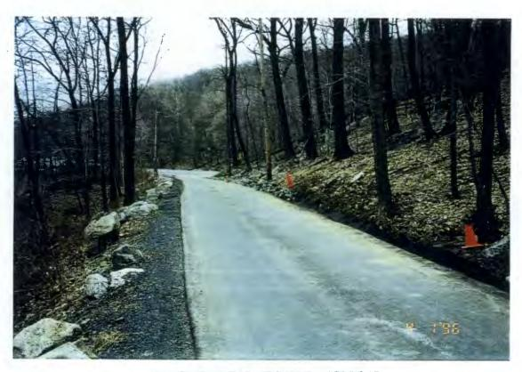
PLACING RIP RAP INTO ENTRANCE ROAD DRAINAGE TRENCH
