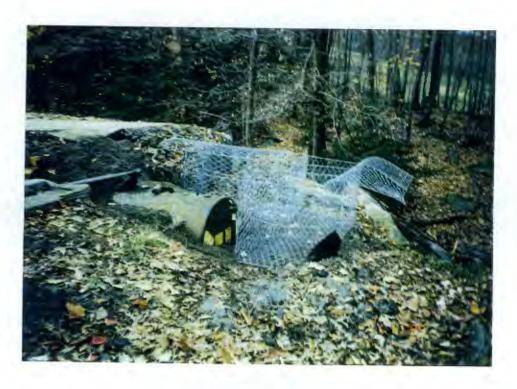
INSTALLATION OF GABIAN BASKET WALL FOR STABILIZATION OF THE TANK
