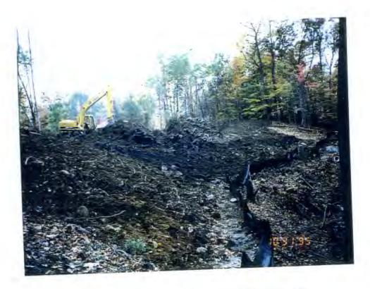
MATERIAL REMOVAL AND SLOPE RE-GRADE
