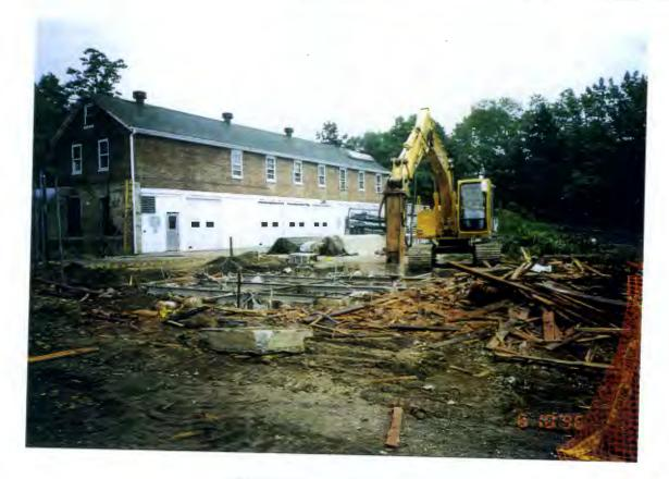
DEMOLISHING THE FOUNDATION OF BUILDING 713A
