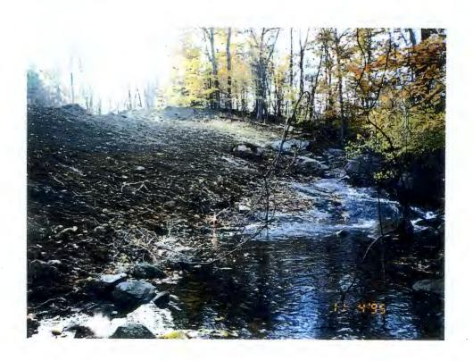
TEMPORARY REMOVAL OF SILT FENCE AND RE-GRADE AT TOE BOUNDARY
