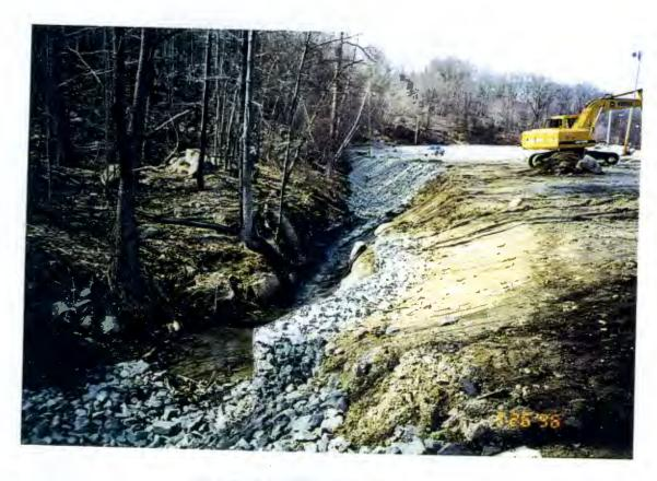
PLACING GEOTEXTILE LINER AND RIP RAP INTO THE DRAINAGE SWALE
