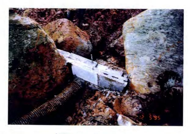
CONSTRUCTION OF COLLECTION BOX AND EXITING SIX INCH PIPE
