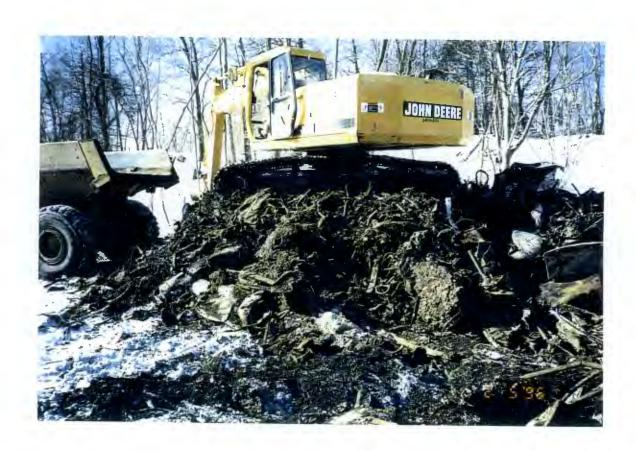
LOADING EXCAVATED LANDFILL MATERIAL INTO ARTICULATED DUMP TRUCK
