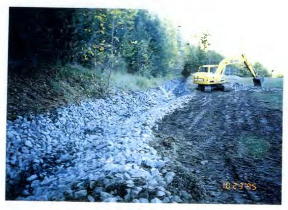
PLACING RIPRAP IN MIDDLE OF THE DRAINAGE SWALE
