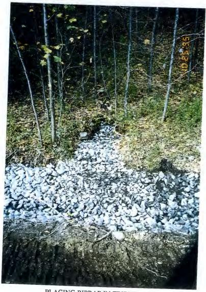
PLACING RIPRAP IN TRIBUTARY ON THE NORTH END OF THE DRAINAGE SWALE
