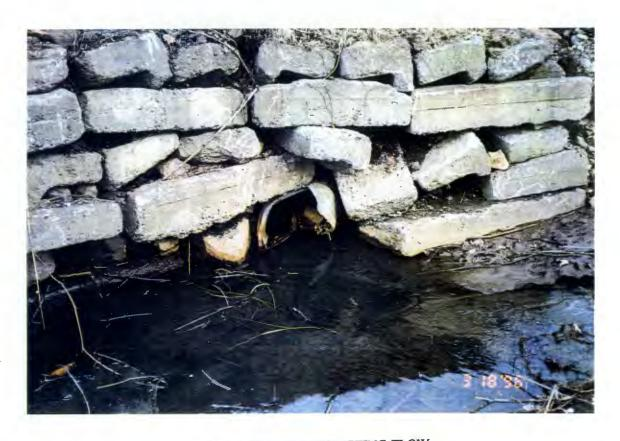
CULVERT BENT IN AND RESTRICTING FLOW
