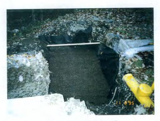
INSTALLED GEOTEXTILE LINER AND PEA GRAVEL FOR BEDDING
