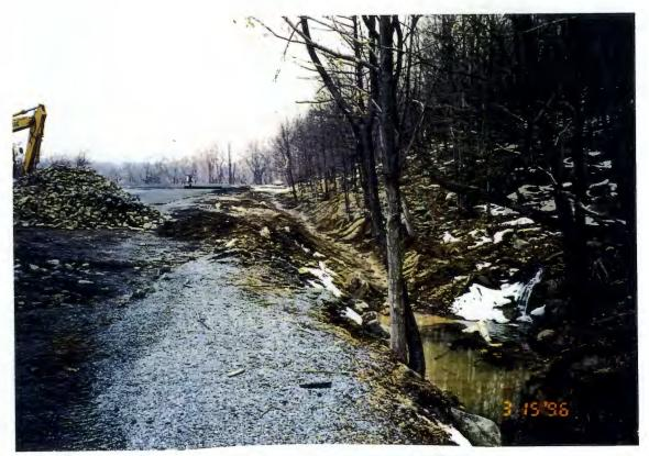
DRESSING THE DRAINAGE SWALE USING THE 690E LC EXCAVATOR
