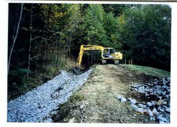
PLACING RIPRAP IN THE NORTH END OF THE DRAINAGE SWALE
