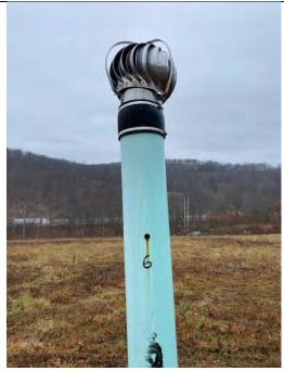
**Photo 4:** View of damaged wind turbine ventilator on GVS-6, looking east.
