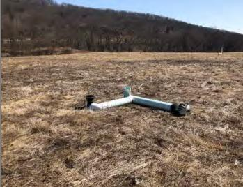
**Photo 3:** View looking southeast at damaged GVS-6 that has completely detached from the base.
