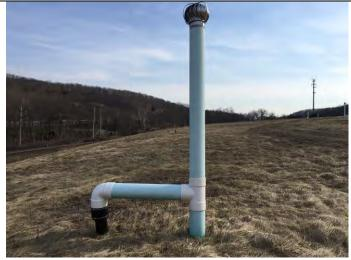
**Photo 8:** Looking southeast. View of gas vent station-1 (GVS-1).
