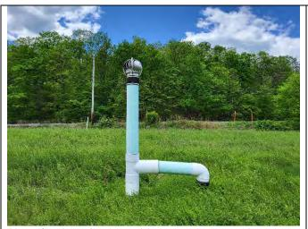
**Photo 9:** View of GVS-6 with damaged wind turbine ventilator, looking west.
