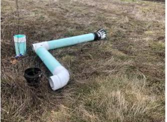
**Photo 4:** Looking downward at damaged gas vent GSV-
