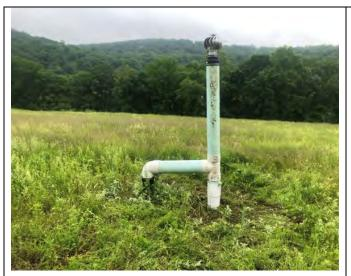
**Photo 5:** Looking east at the repaired gas vent, GVS-11.
