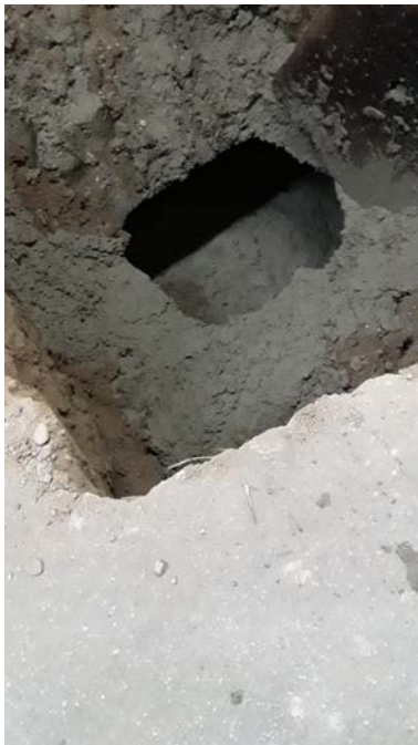
Filling tank with concrete
