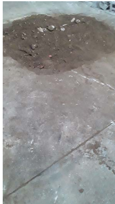
Surface restored to grade
