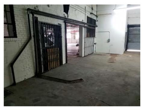
5. Fill and vent lines showing the area of 2,000-gallon fuel oil underground storage tank (UST), located at southern-central portion of warehouse
