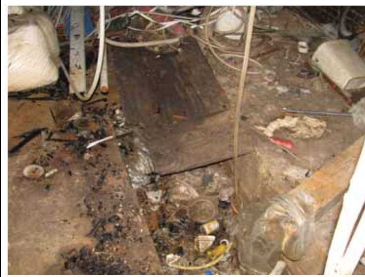
Garbage filled trenches and drains inside of the building.
