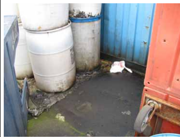
Heavy staining and residual slime associated with drums next to the shipping containers.
