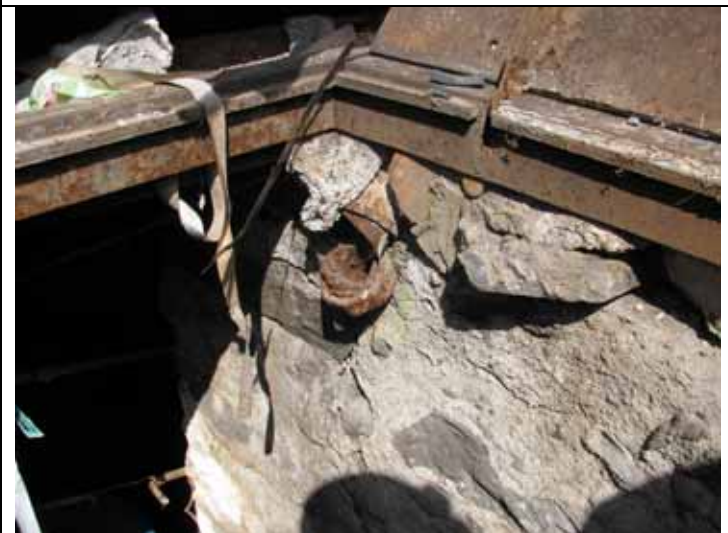
Cut piping believed to be former AST/UST fill piping.
