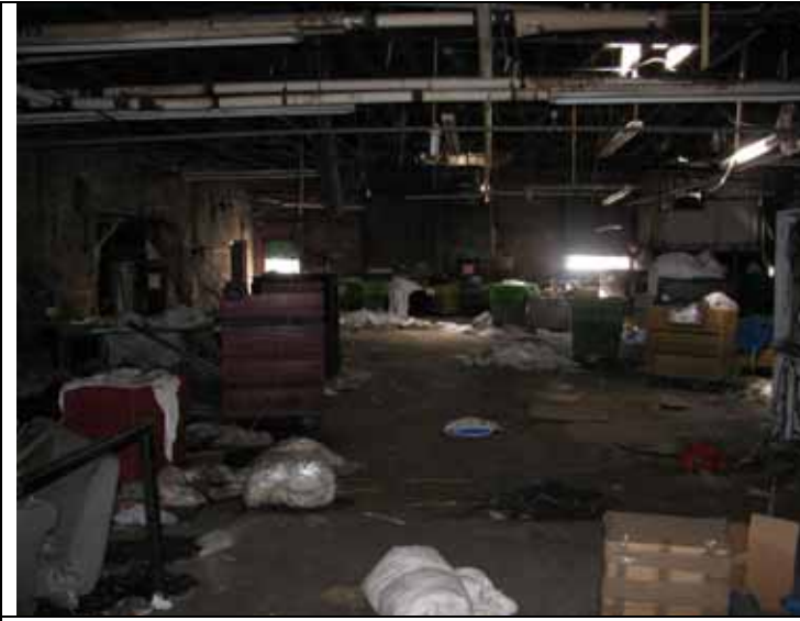
Interior of southern portion of building.
