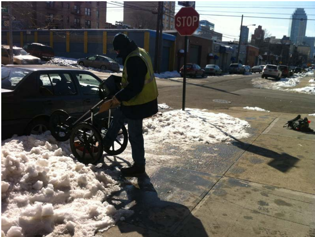
Utility Check February 11, 2014
