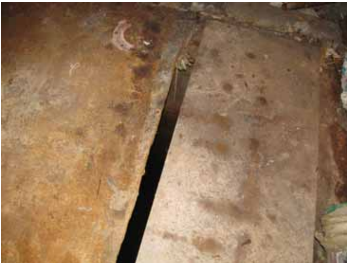
Steel road plates over sump.
