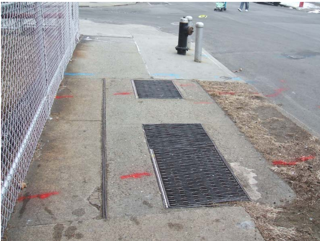
Utility Clearance – Lines Running from 37-24 24 th Street Equities to 38 th Avenue February 7, 2009
