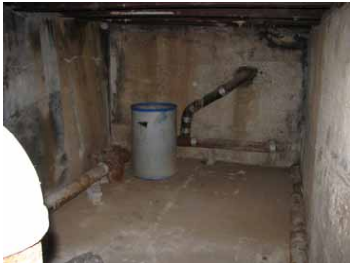
Southern basement interior.
