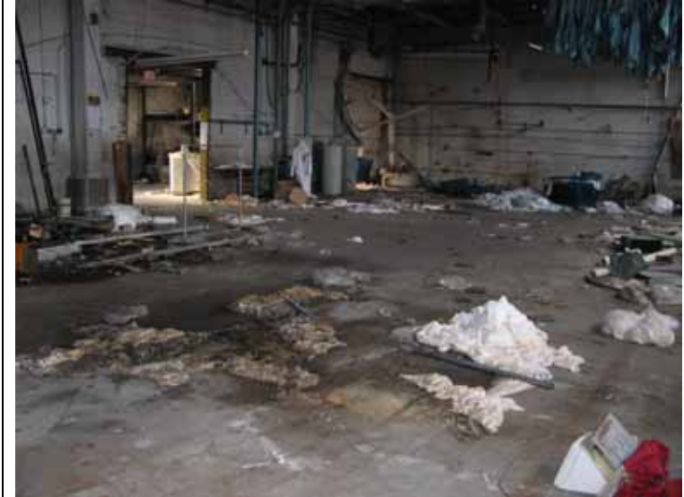
Interior of northern portion of building
