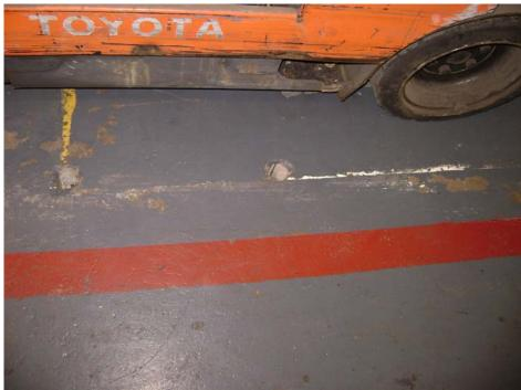
Photo #90: Holes in subslab.
