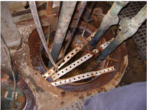
Photo #11: Sump #1, collected water sample via bailer.
