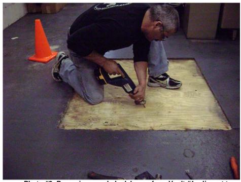
Photo #2: Removing wood plank layers from Vault #1 adjacent to MW15.
