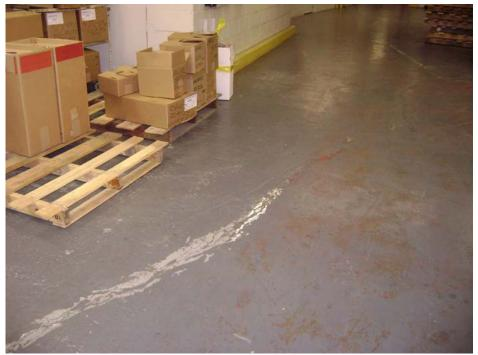
Photo #91: Thin crack in subslab within the faded painted area.
