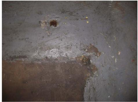
Photo #89: Holes in subslab.
