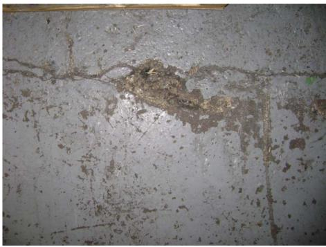
Photo #92: Cracks in Subslab.
