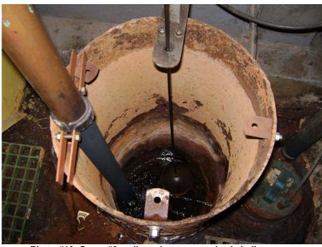
Photo #10: Sump #2, collected water sample via bailer.
