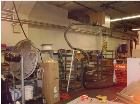
Photo #50: Venting fumes of Geoprobe rig while drilling inside.
