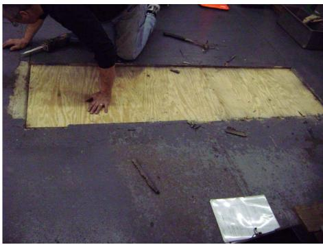
Photo #6: Removing wood plank layers from Vault #2.
