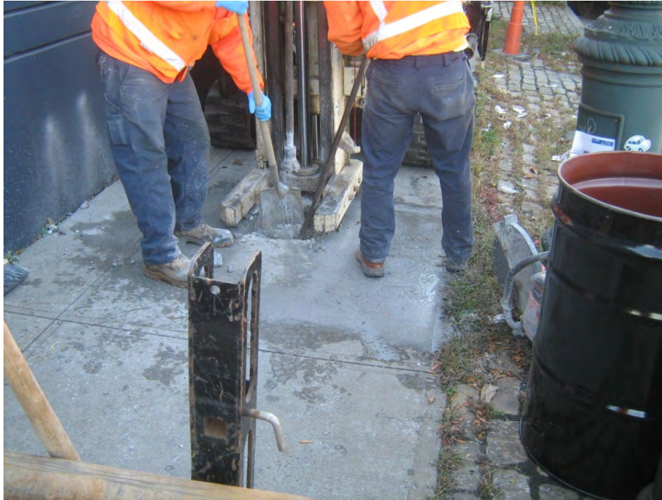
Photo 9: Completion of soil boring location SB-05 by Geoprobe.
