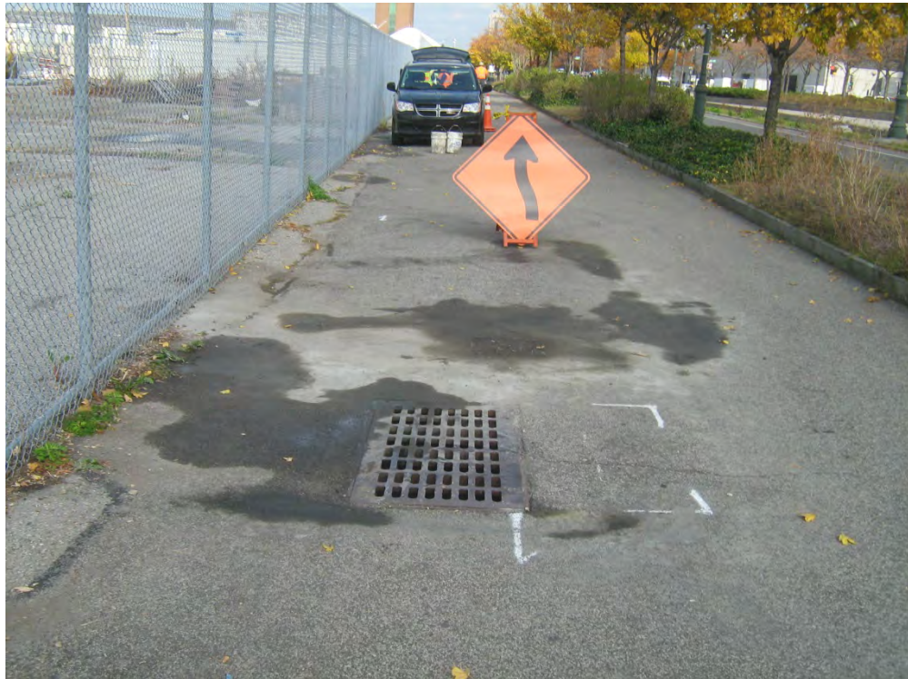
Photo 12: Soil boring location SB-09 after soil boring completed, looking north.
