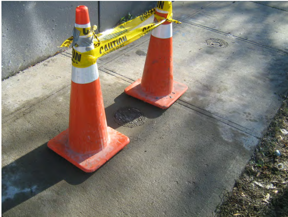
Photo 16: Completed groundwater monitoring well DBMW-01.
