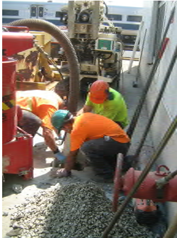
Photo 5: Hand clearing at soil boring location SB-08.
