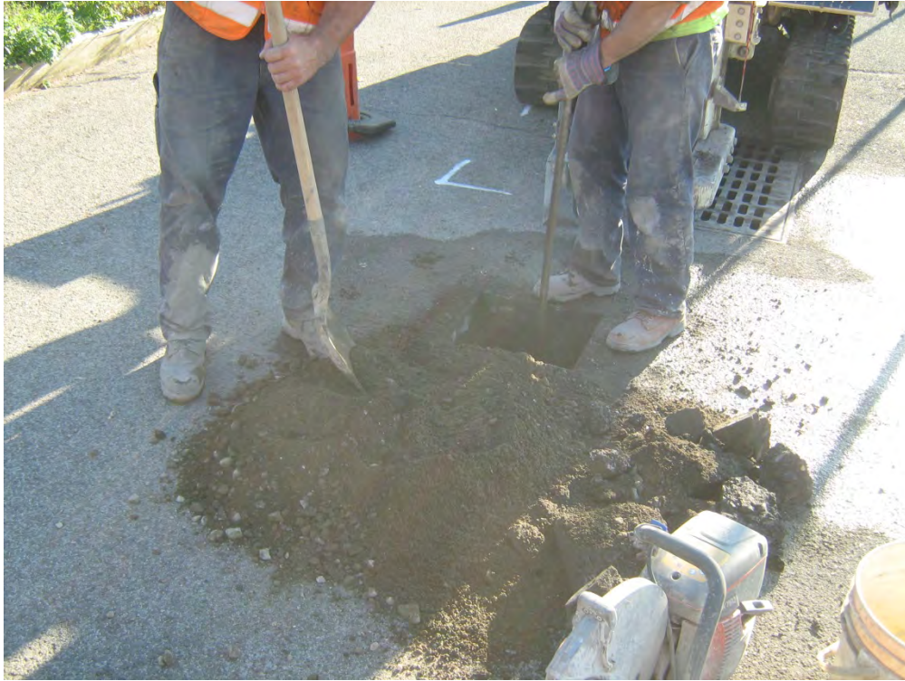
Photo 11: Hand clearing at soil boring location SB-09.
