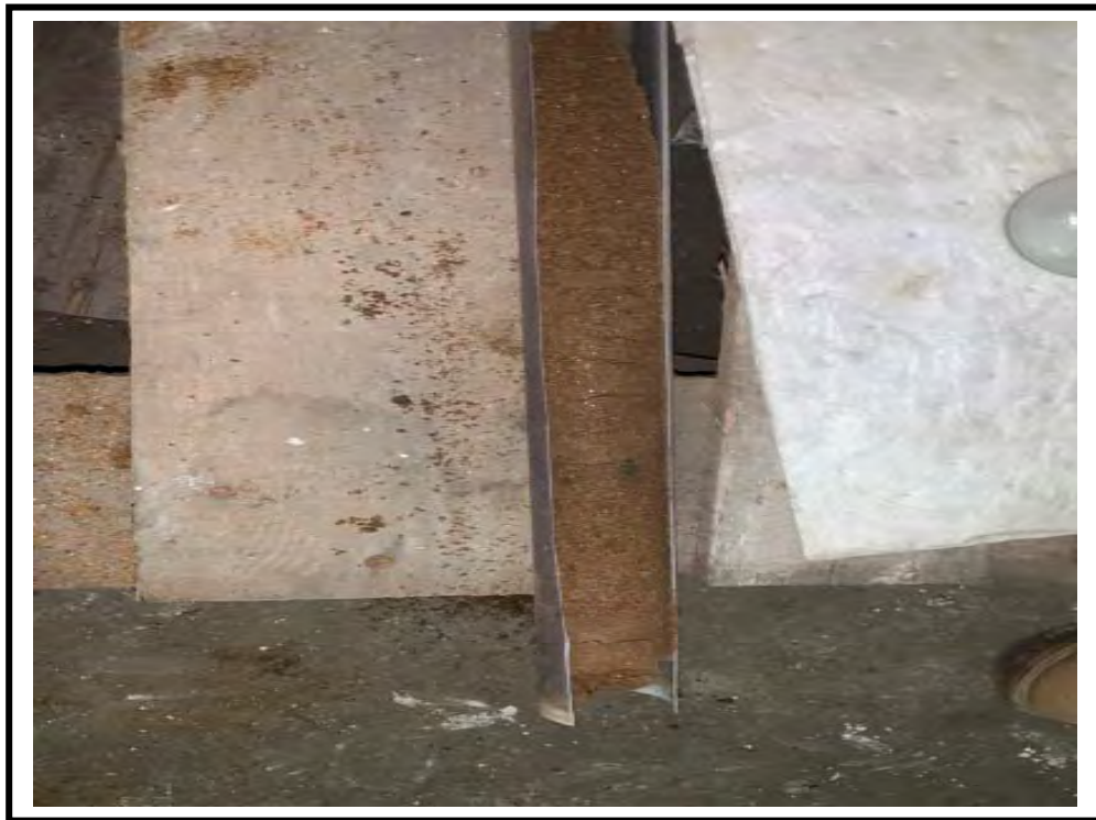
PHOTO LOCATION: Depicts the coring for SB-3.
