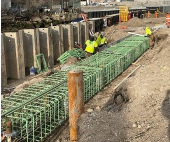
Figure 1: Installation of rebar for deadman at DSNY Salt Lot
