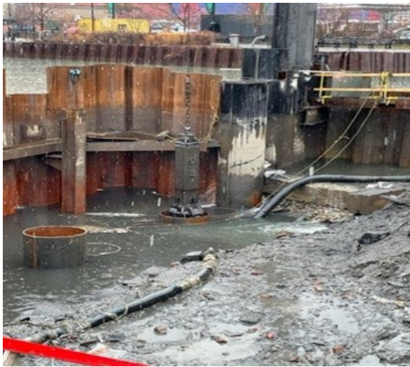
Figure 2: Cleaning inside of pipe piles at DSNY Salt Lot
