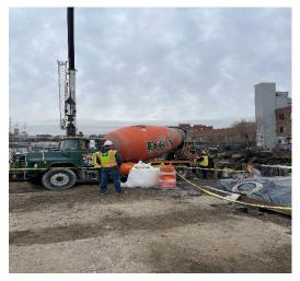
Figure 7: Pouring concrete in pipe piles at DSNY Salt Lot
