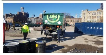
Figure 2: Removing drum with soil from UST bottom
