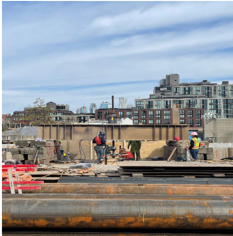
Figure 6: Setting up for load test at DSNY Salt Lot
