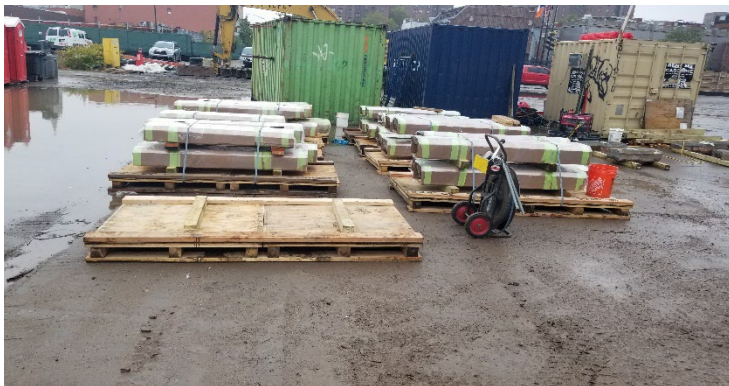
Figure 1: Packed bluestone watertables for offsite shipment
