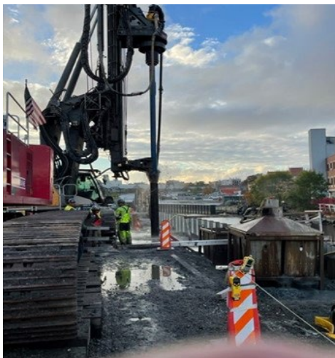
Figure 4: Drilling of tensile test rig at DSNY Salt Lot
