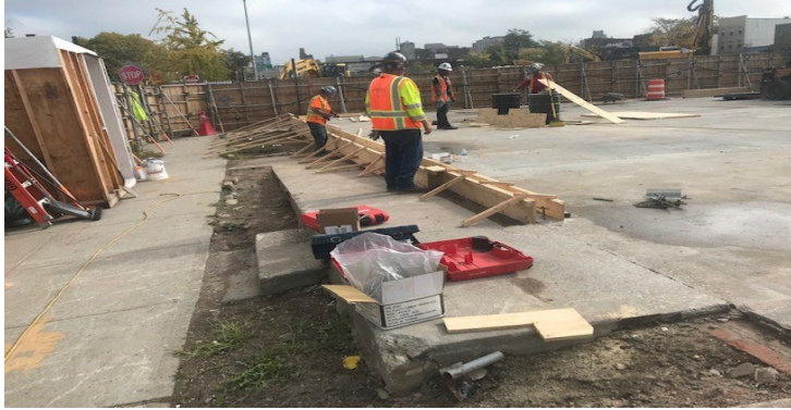
Figure 3: Formwork for perimeter curb at 270 Nevins St.
