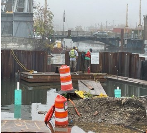
Figure 5: Cutting windows in coffer dam at end 2 nd Ave.
