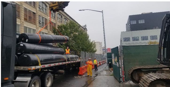
Figure 2: Delivery of Geomembrane for 270 Nevins St.
