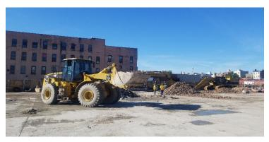
Figure 4: Clearing debris from demolition at 270 Nevins St.
