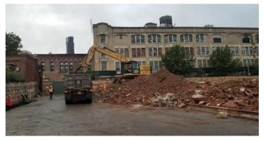
Figure 1: Loading out debris from 234 Butler St.
