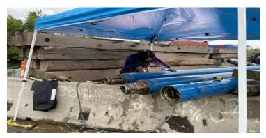
Figure 7: Welding of centralizers on drill steel at DSNY Salt Lot
