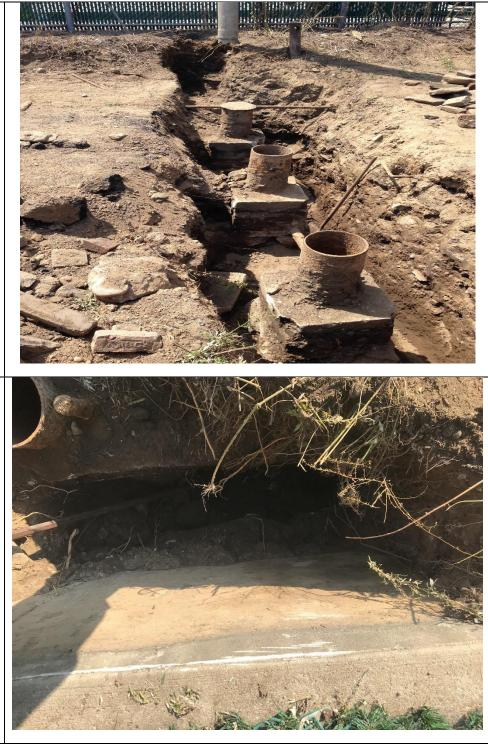
Photo 6 – Top westernmost valve port and fill or vent pipe on southern side of UST-1 area near site boundary fence and Vandervoort Avenue. Tank is accessible through small pipe visible in photo. Top of concrete vault approximately 4 feet below the top of the valve port.
