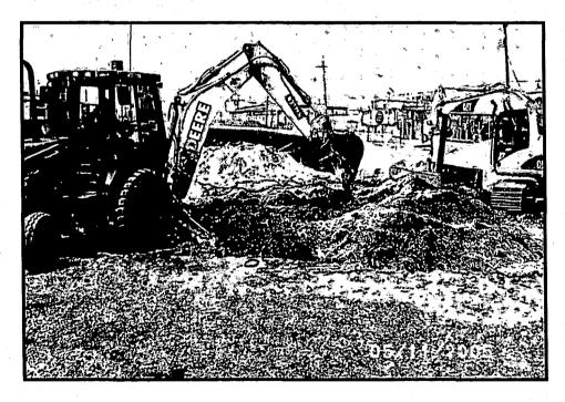
Excavation Area B – Excavation of impacted soils; use of odor suppressant foam
