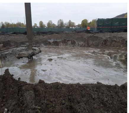
ISS is an established remediation treatment technology used to prevent migration of and exposure of MGP contaminants in media including soil.
