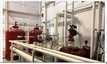
500-gal Ansul tanks connected to the deluge system (top) and hangar drain leading to the underground storage tanks (bottom).
