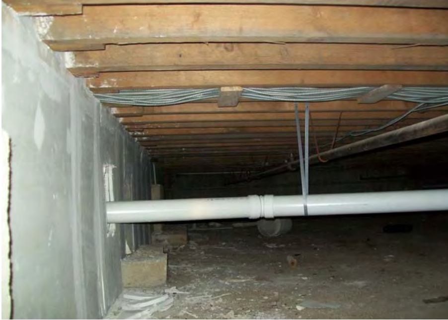
5. Suction piping at western side of drywall partition, looking south
