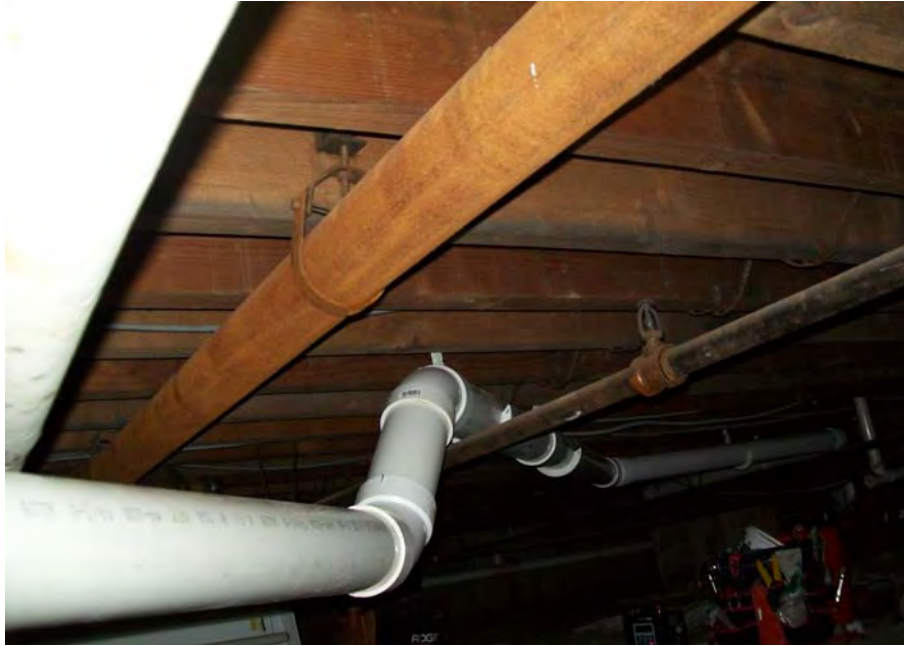
7. Suction piping, looking southwest from near MP-1 toward crawlspace entrance
