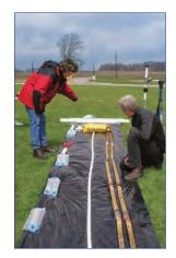
Installation of a 3-Channel CMT System with bentonite and sand cartridges. Three zones were monitored over a 20 ft (6 m) depth. The installation was completed in glacial till at the University of Waterloo, Ontario Canada.
