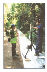
CMT System installed to a 60 m (200 ft) depth with seven monitoring zones. Installation was completed by placing layers of sand and bentonite to monitor a BTEX/MTBE plume in a Chalk aquifer, United Kingdom.
