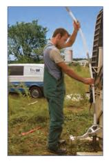
3-Channel CMT installation at a plant in Zeitz, Germany. Systems were completed using natural collapse and are being used to assess natural attenuation of BTEX.
