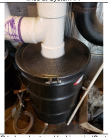
PVC to knockout seal leaking air. (System #1)
