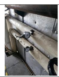
Pressure gauges installed in PVC influent lines at System #1
