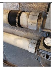
Fernco coupler loose and missing hose clamp at System #1.
