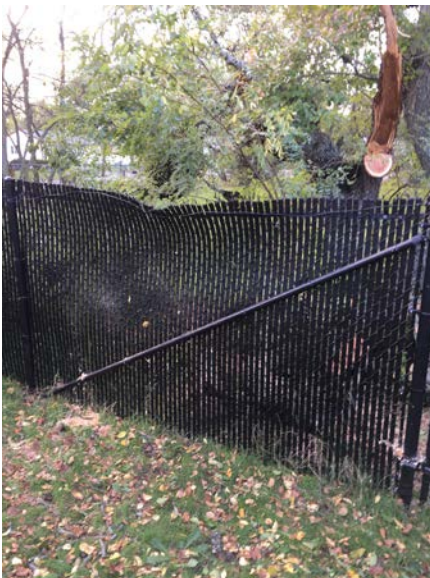
Damage to fence from tree
