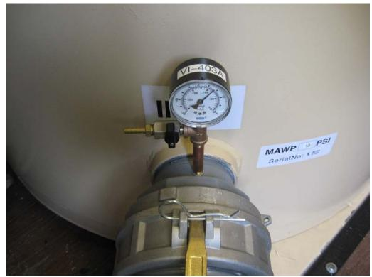
Carbon vessel vacuum gauge and sampling port. NOTE: white tag on right displays Maximum Allowable Working Pressure (MAWP) at 10 psi.
