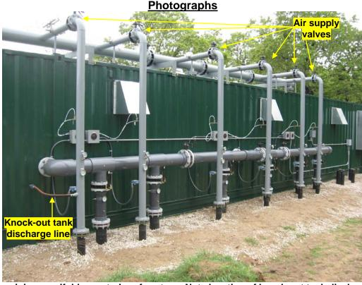
View of air-line piping manifold on exterior of system. Note location of knock-out tank discharge line and air supply valves.
