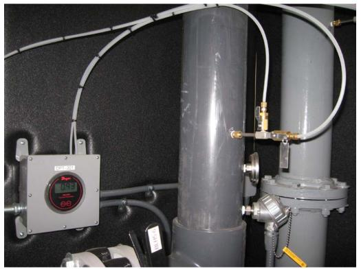
View of digital pressure transmitter and associated pitot tubes.
