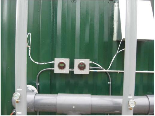
View of two digital pressure transmitters monitoring air supply pipes.
