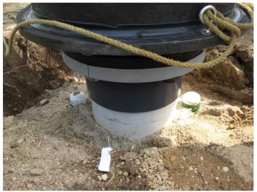
Close up view of DDC-05 well head and PVC well casing connection.
