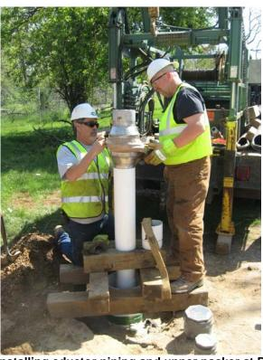
Layne installing eductor piping and upper packer at DDC-05.
