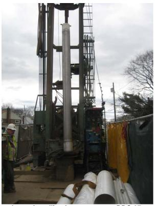
Layne installing lower screen at DDC-07.
