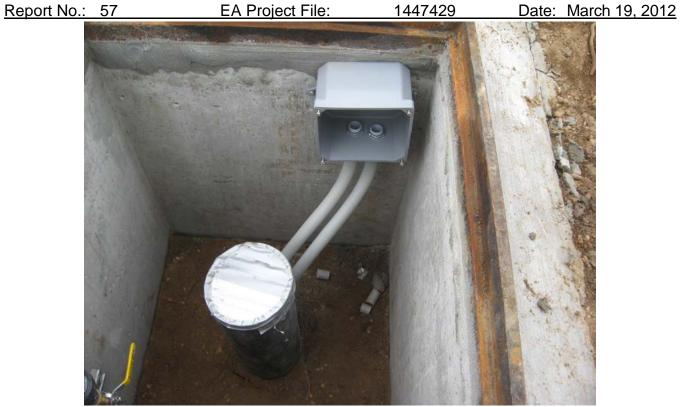
View of electrical box partially installed in sump vault.
