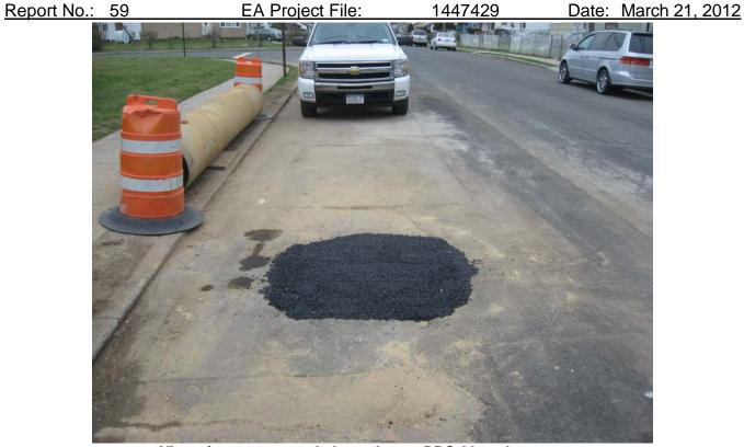
View of temporary asphalt patch over DDC-08 vault man-way.
