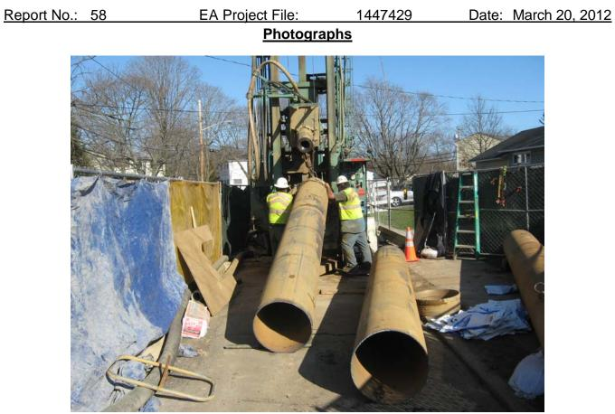
Layne removing outer casing at DDC-08.
