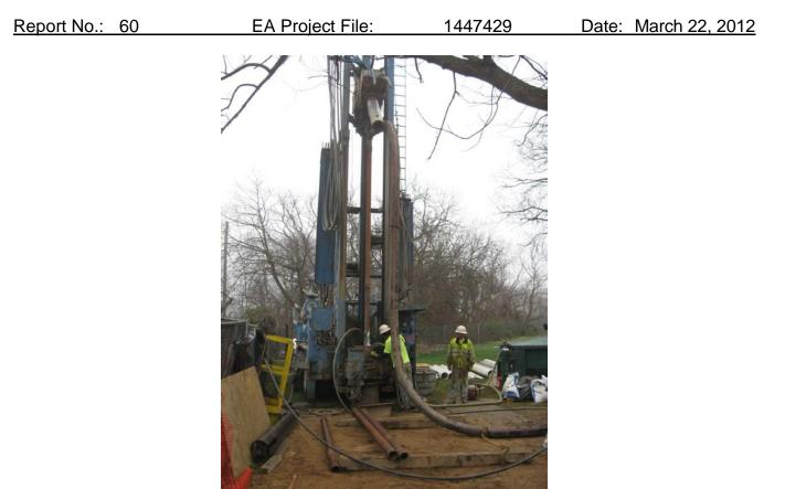
View of Layne bailing sediment from DDC-05 borehole.
