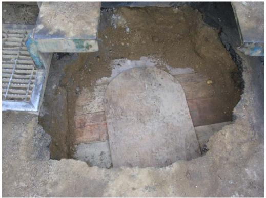
Timber used to seal DDC-08 man-way.
