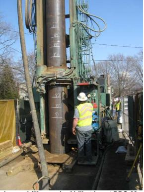
Layne drilling casing/drill string at DDC-08.
