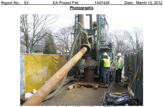
Layne threading additional drill rod at DDC-08.
