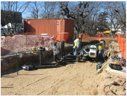
View of air lines being installed along north side of treatment system pad.
