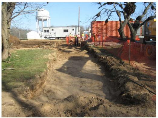
View of partially backfilled trench line to treatment system pad, looking east.
