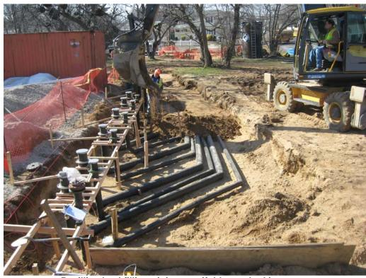
Posillico backfilling piping manifold area, looking west.
