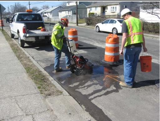
Posillico saw-cutting temporary asphalt patch at DDC-08.
