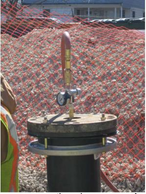
Close up of air compressor connection and pressure gauge for pressure testing.
