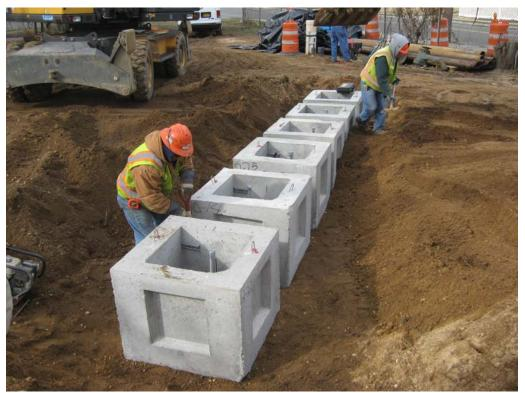
View of concrete sump vaults being installed.
