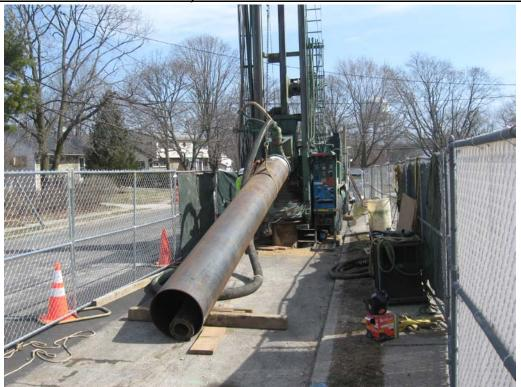
Layne attaching 24-in. diameter outer casing at DDC-08.
