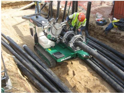
View of Posillico connecting piping in trench line via heat fusion.
