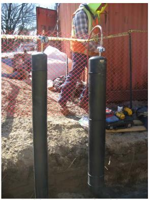
Posillico pressure testing piping.
