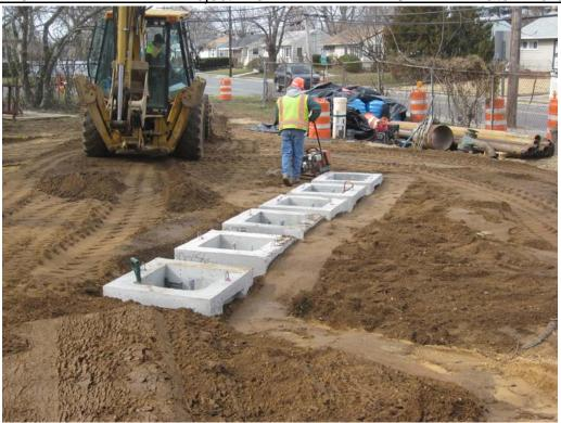
Posillico backfilling/compacting sump collection area.
