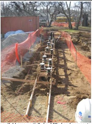
View of piping manifold area partially backfilled and compacted, looking west.
