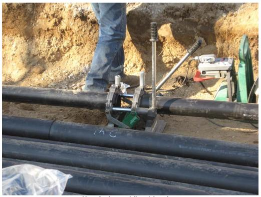
Heat fusion welding 4-in. pipe.
