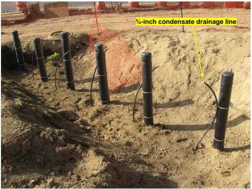
View of 3/4-in. condensate drainage lines in sump collection area.
