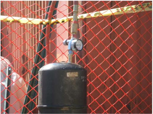
Close up of air compressor connection and pressure gauge on HDPE piping.
