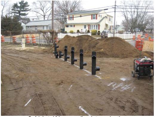
Prefabricated 6-in. sumps aligned at sump location.
