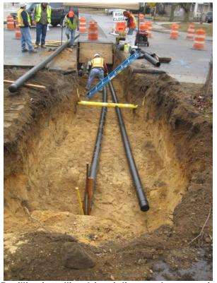
Posillico installing 6-in. air lines under gas main.
