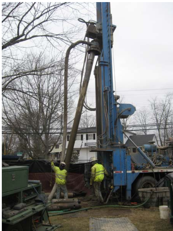
Layne inserting additional drill rods into DDC-05.
