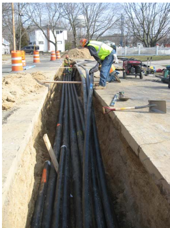
View of piping in trench line, looking east.
