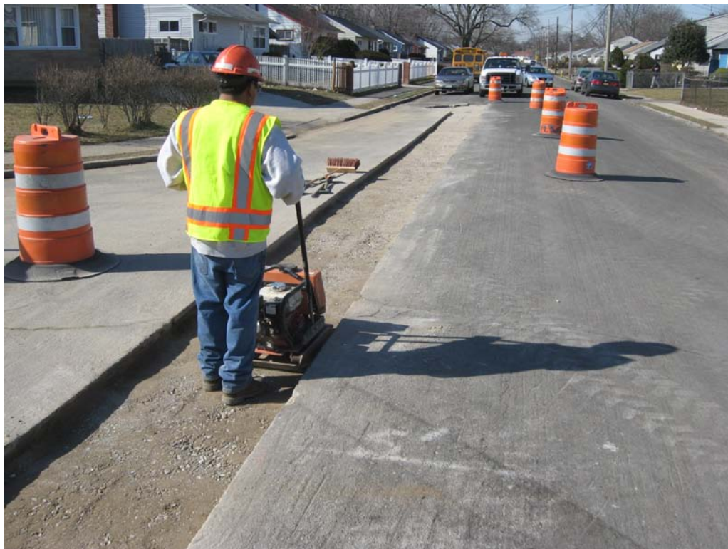
Posillico compacting sub-base with plate compactor.
