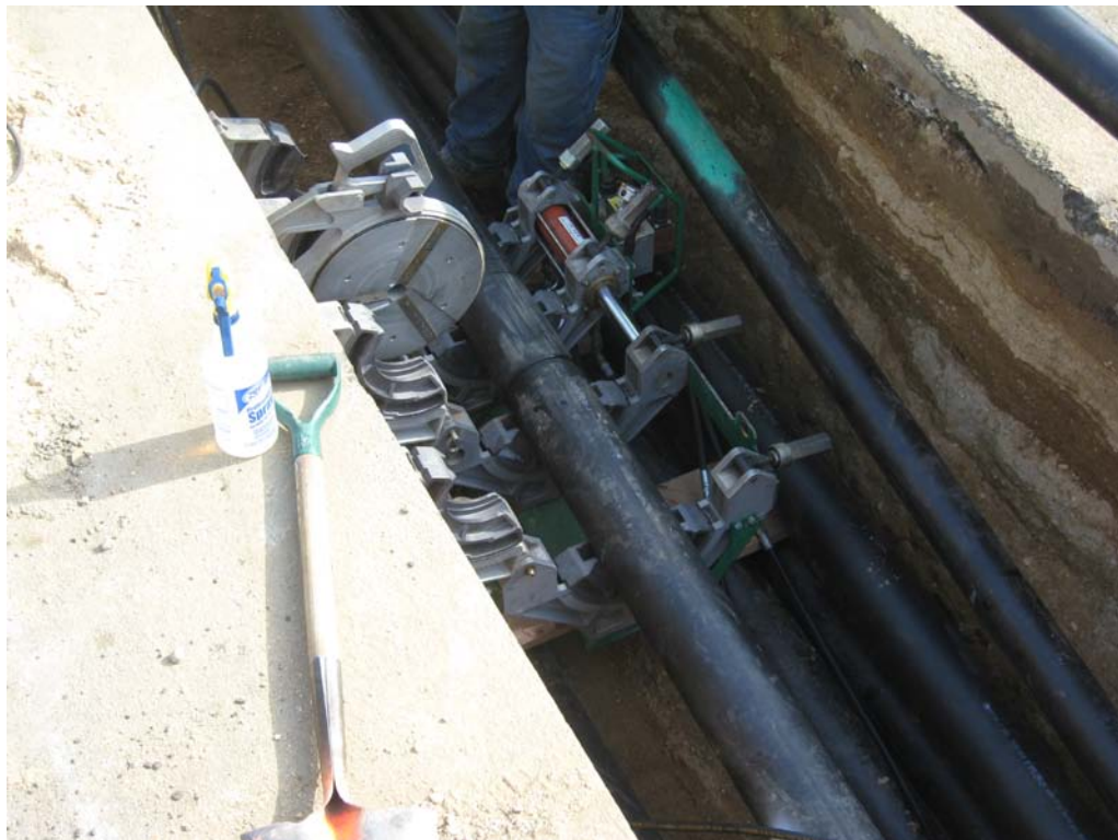
Heat fusion weld being performed in trench line.
