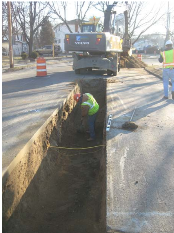
Posillico trenching between DDC-08 and DDC-07, looking east.
