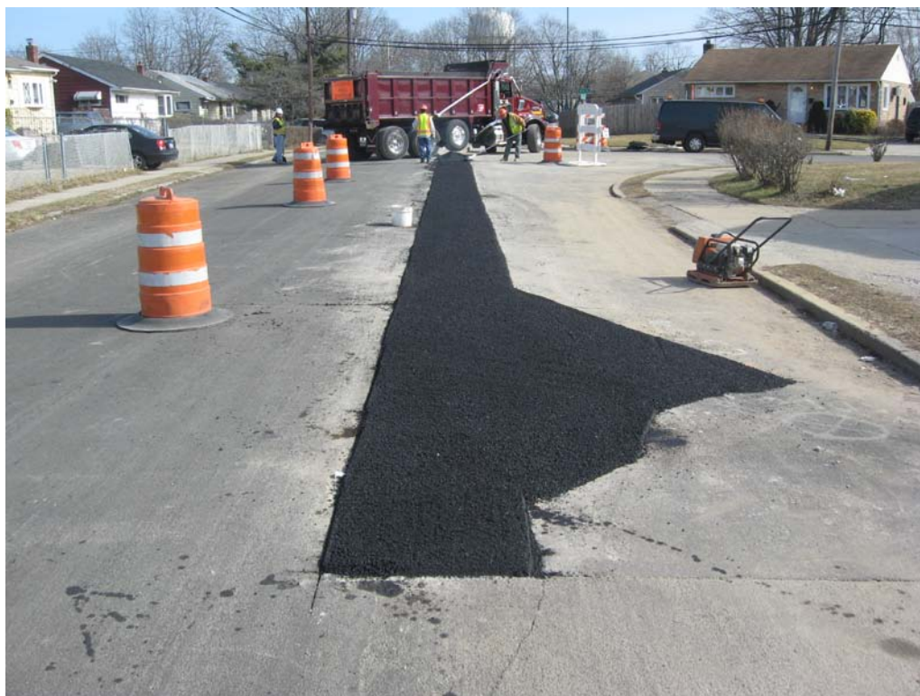
View of temporary asphalt at DDC-10 looking east.
