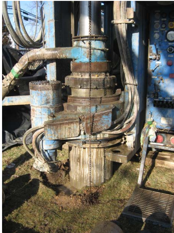
View of 24-in. outer casing at DDC-05.
