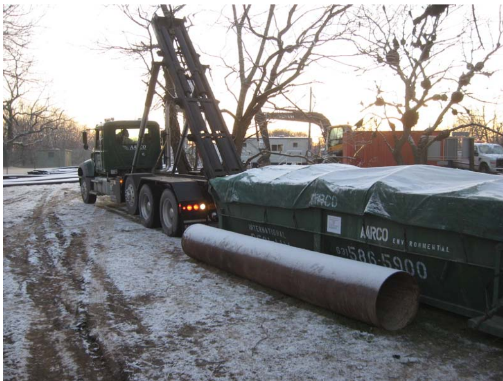
Aarco loading roll-off for off-site disposal. Contents: DDC-06 drill cuttings.
