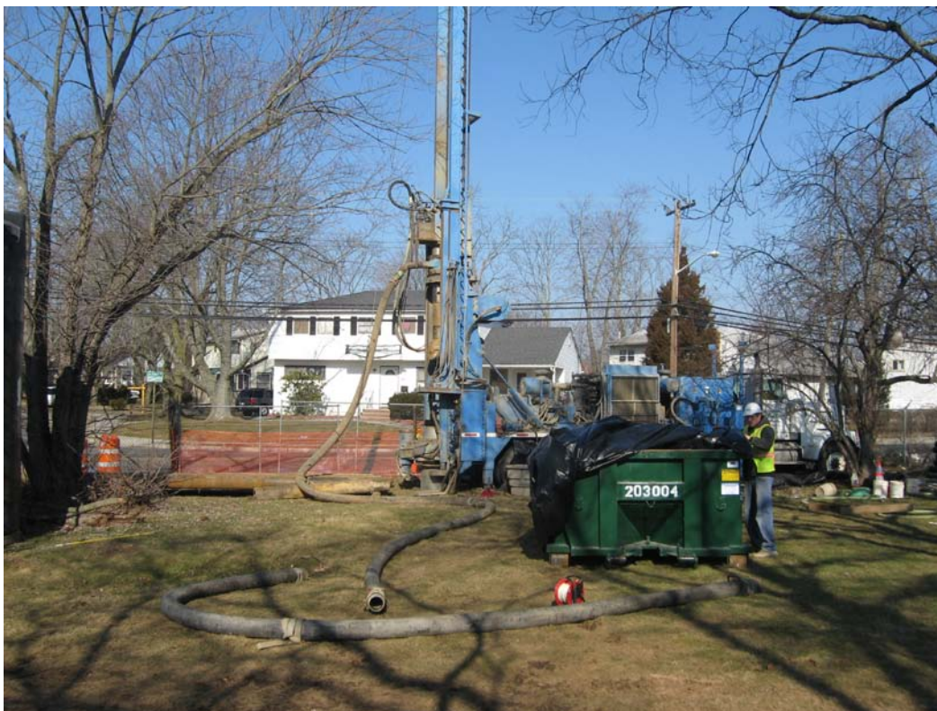
Layne at DDC-05 and poly lined roll-off, looking northwest.
