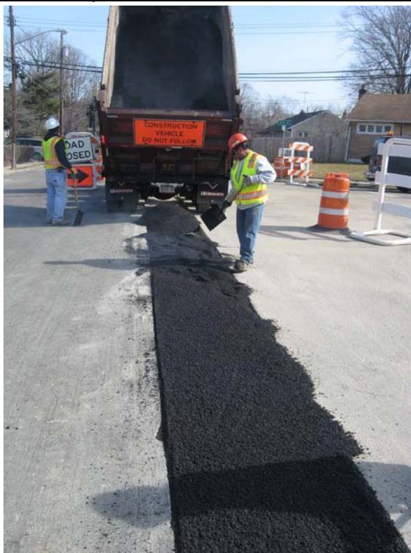
Posillico placing temporary asphalt from DDC-10 to DDC-09, looking east.
