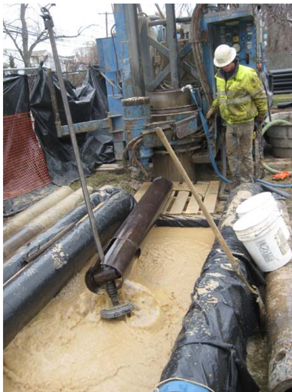
View of Layne removing material via bailer.
