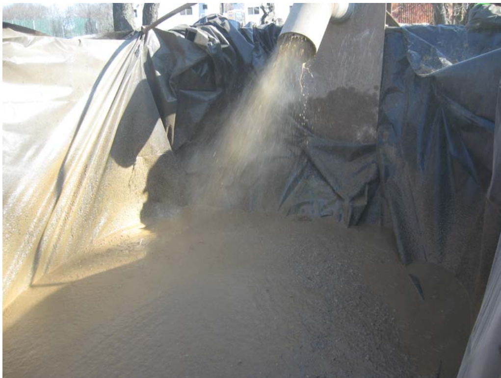
Drill cuttings and water being ejected into poly lined roll-off.
