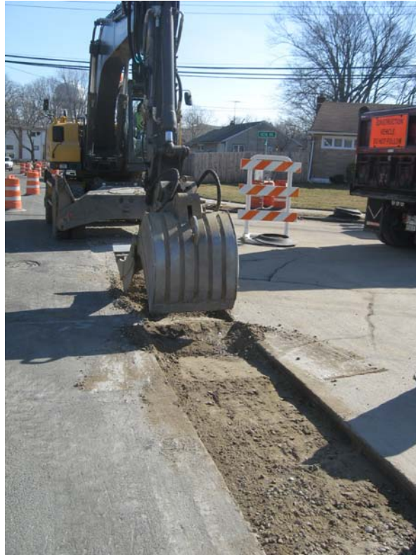
Posillico removing 4-in. of recycled concrete to accommodate asphalt.
