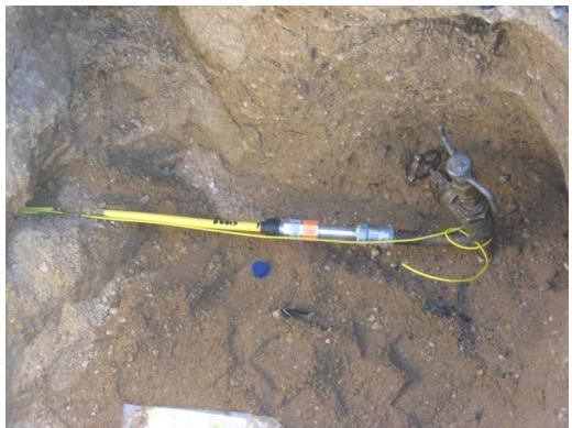
View of replaced 1 in. gas line at 4 in. main connection point.
