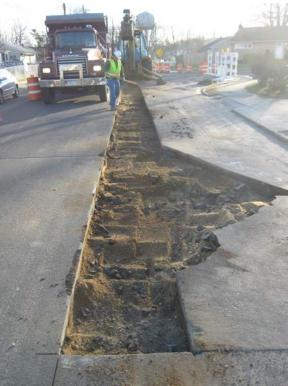
Posillico removing asphalt from trench line, at DDC-10 looking east.
