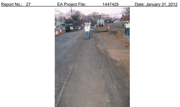
Posillico compacting crushed concrete at grade for road use.
