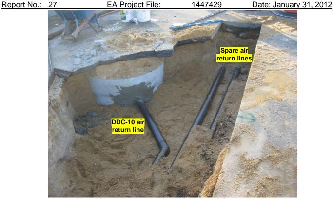
View of 4 in. return lines at DDC-10 (one at DDC-10, two spares).
