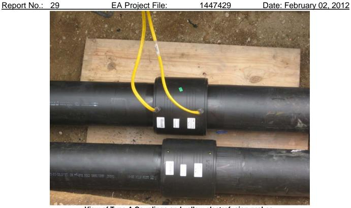
View of Type A Couplings and yellow electrofusion probes.
