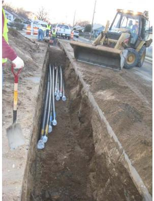
HDPE air lines extending through trench line, at DDC-08 looking west.
