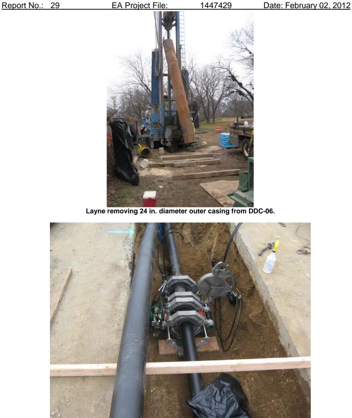
Posillico performing heat fusion weld in trench.
