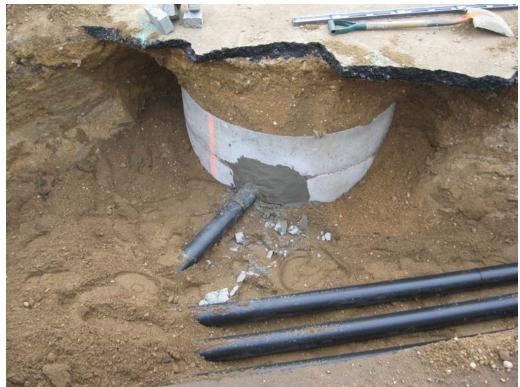
View of 4" air line attached to DDC-08 vault.
