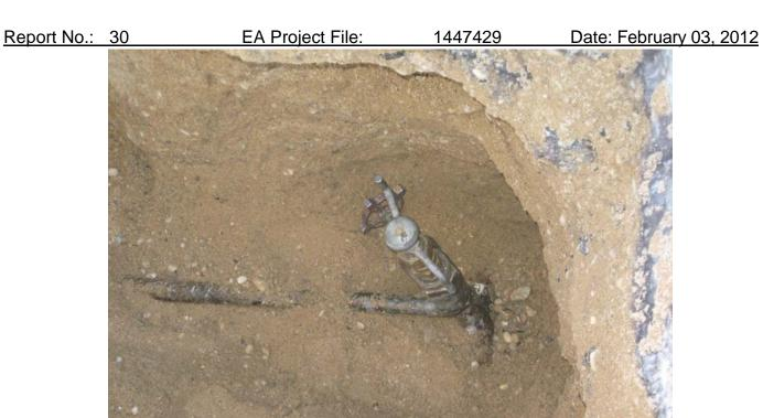
View of 1 and 4 in. gas line connection points with shut off valve.
