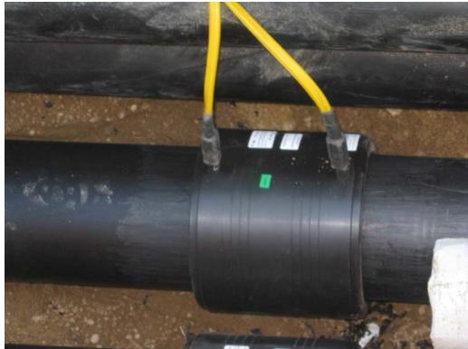
View of Type A Coupling and yellow electrofusion probes.
