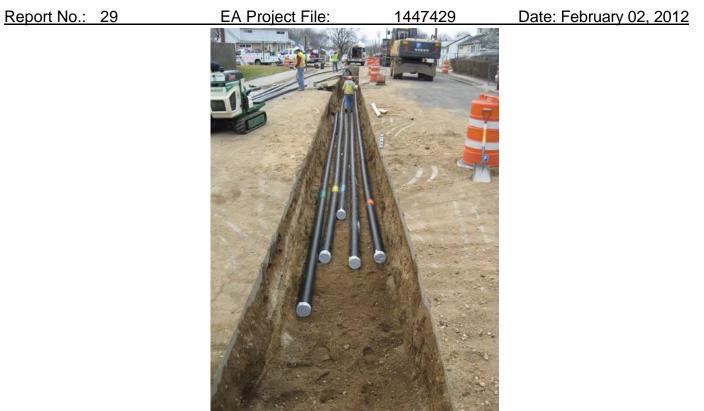
HDPE air lines extending through trench line, at DDC-07 looking west.
