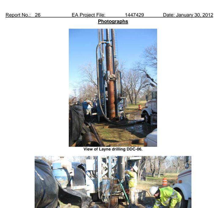
Layne using 6-in. diameter bailer to remove sands.
