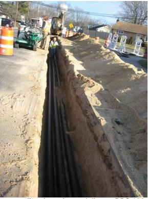
HDPE piping extending through trench line, at DDC-10 looking east.
