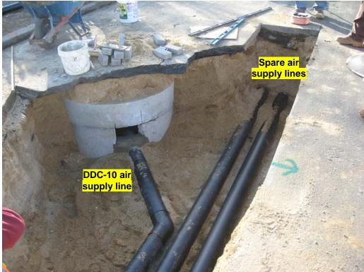
View of 6 in. supply lines at DDC-10 (one at DDC-10, two spares).
