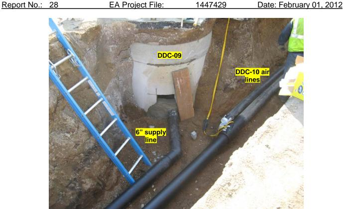
View of 6 in. air supply line inserted into DDC-09 vault.
