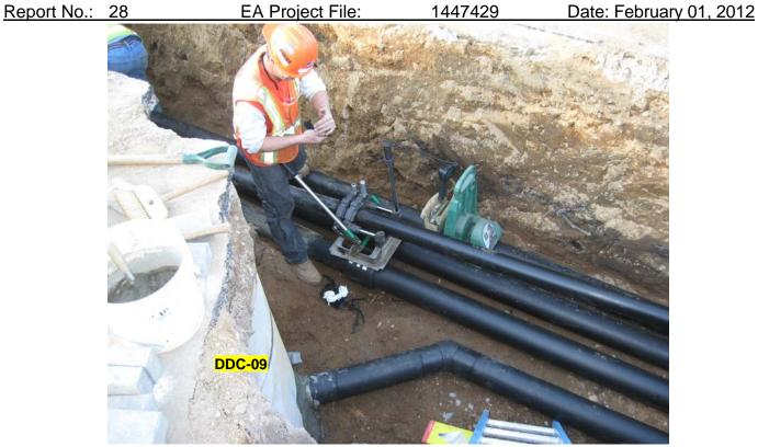
Posillico performing heat fusion weld in trench.
