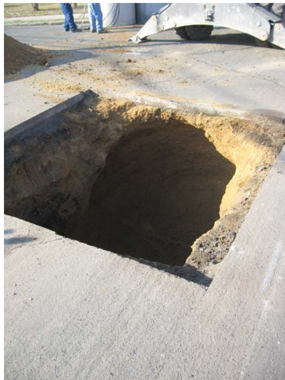
View of DDC-09 excavated area.
