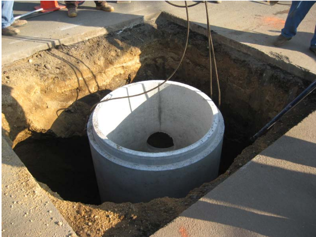
Installation of manhole casing/vault.
