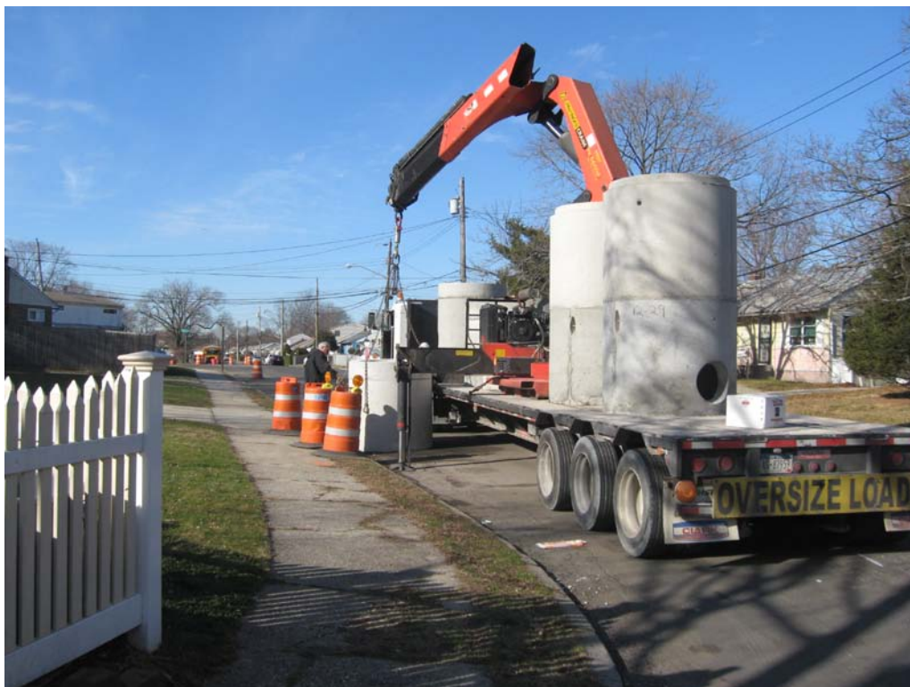
View of Posillico unloading precast concrete casings.
