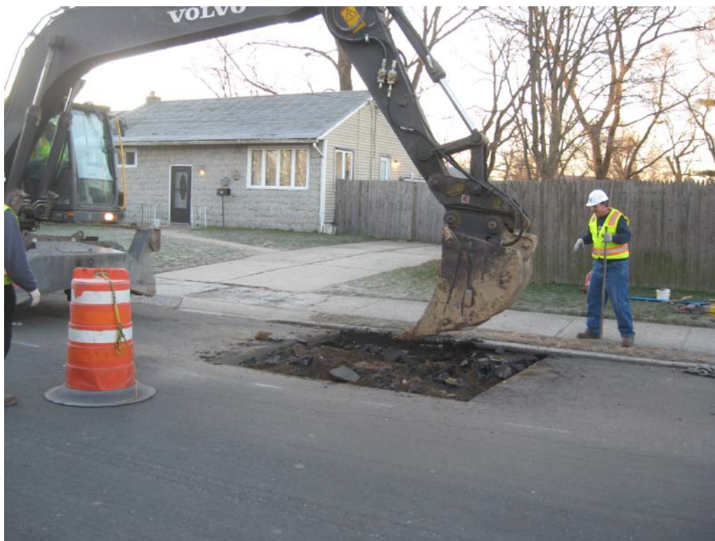
Posillico removing asphalt at DDC-08.
