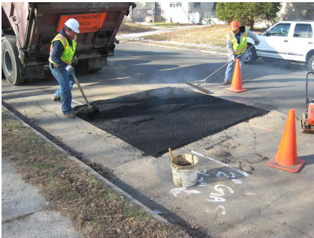
Posillico placing temporary asphalt patch at DDC-07.
