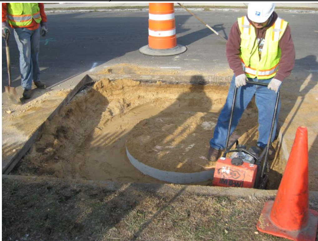
Compacting backfill around casing.
