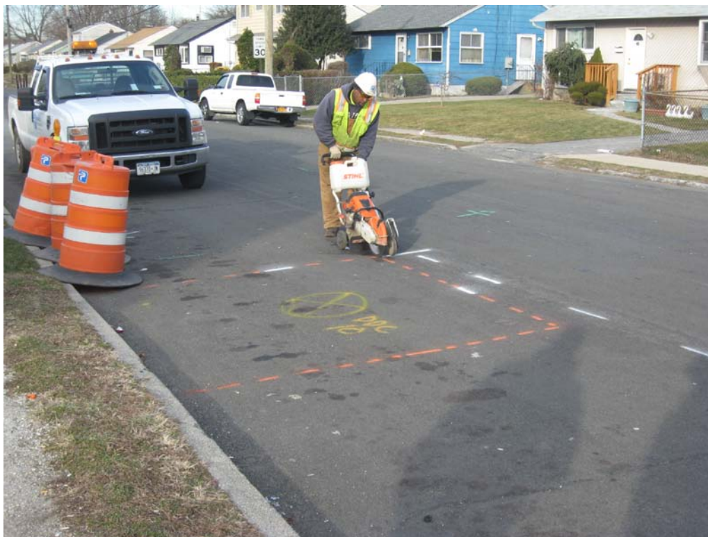
Posillico saw-cutting DDC-10.
