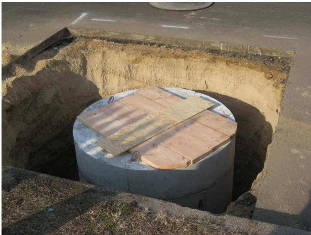
Lumber used to seal opening to casing before backfilling.
