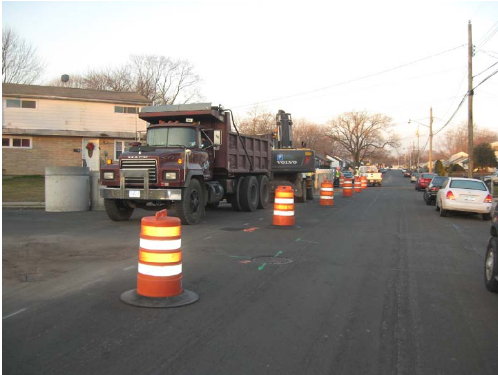
View of traffic controls and general setup.
