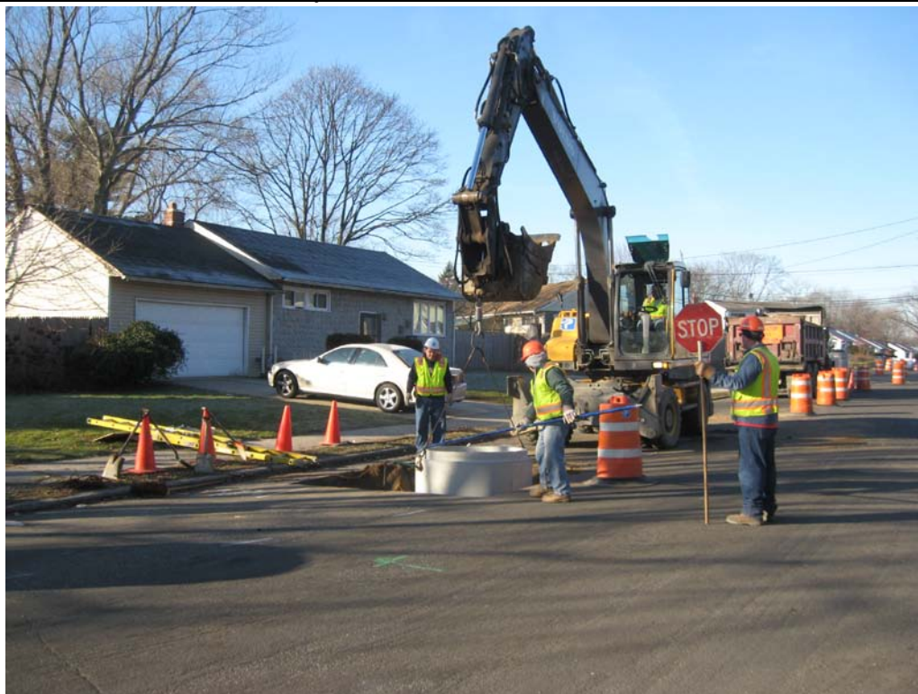
Installation of manhole casing/vault at DDC-07.
