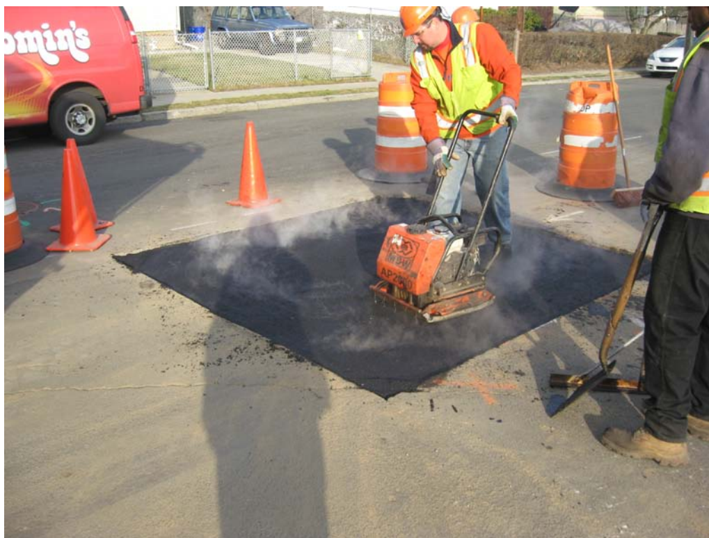
Compacting temporary asphalt patch.
