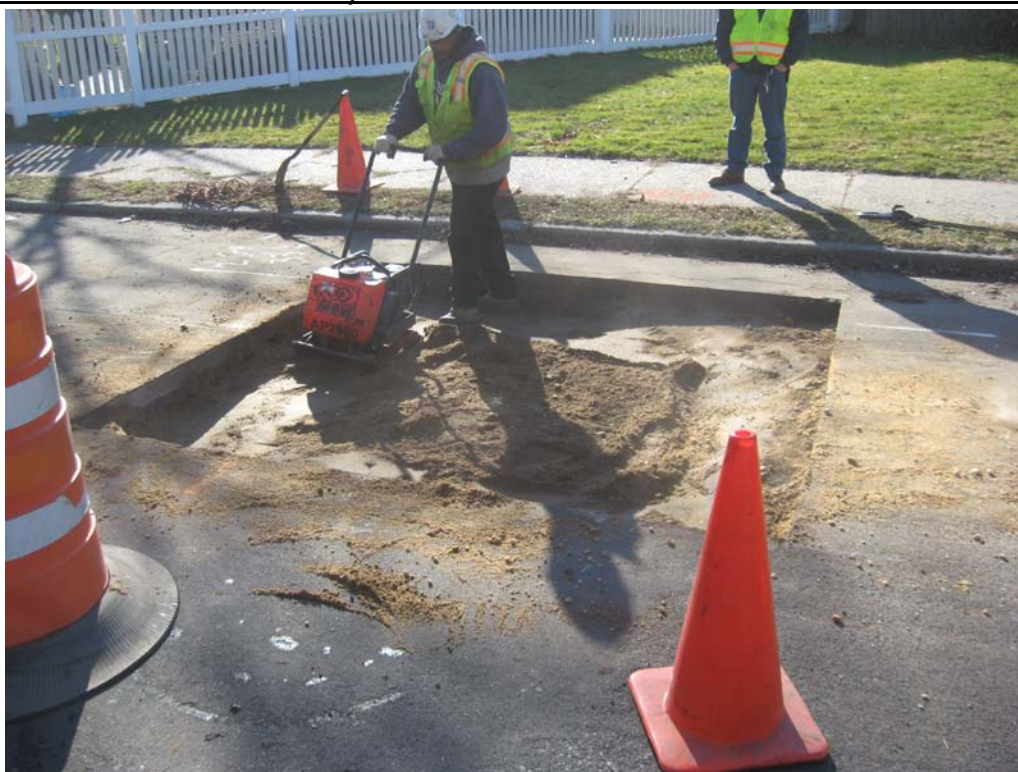
Compacting backfill around casing.
