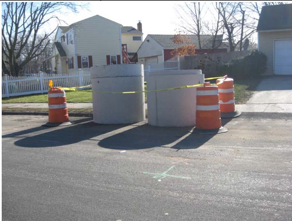
View of casings staged along Benjoe Drive.
